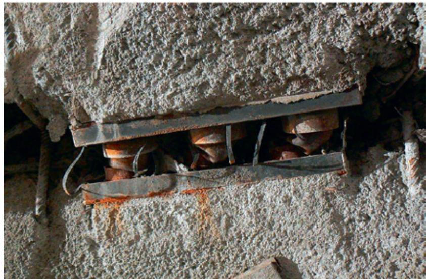
Abb. 5. Stauchelemente LSC | Fig. 5. LSC lining stress controllers
