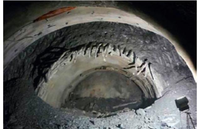
Fig. 3. Excavation and Support Type 7C
