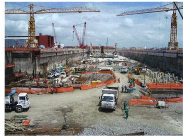
Construction underway for the dock floor
