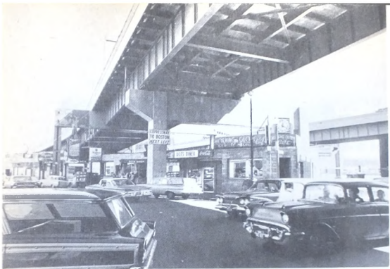
Elevated highway of today
