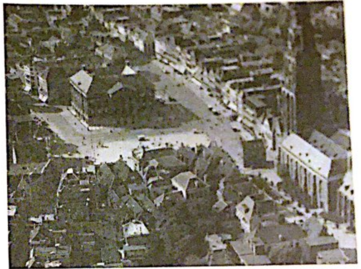
FIG. 66: Air view of Groningen. The three-dimensional emphasis of the church tower signals the presence of both the quiet churchyard garden to the right and the busy town hall square to the left.
