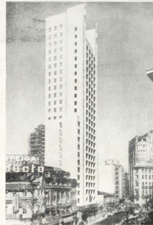
Serious settlement of a corner of this tall concrete building was recovered by jacking it onto new piers sunk through artificially frozen sand.
