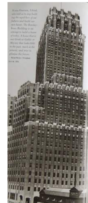
Fig.38 Barclay-Vesey Building, NY, 1926. DUPRÉ, 1996, p.34.
