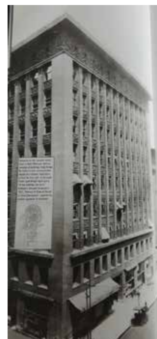
Fig.31 Wainwright Building, Adler & Sullivan, St. Louis, Missouri, 1891. DUPRÉ, 1996, p.21.
