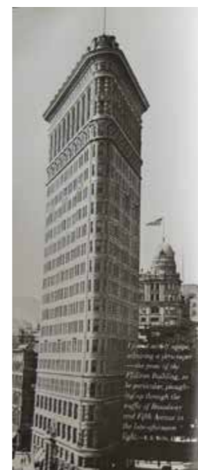
Fig.34 Flatiron Building, NY, Daniel Burnham, 1902. DUPRÉ, 1996, p.24.
