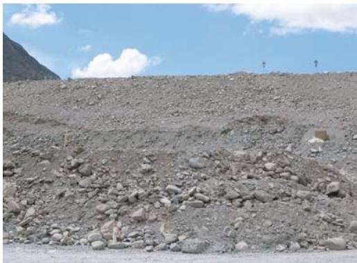
Fig. 2 Rockfill dam – Caracoles Dam
