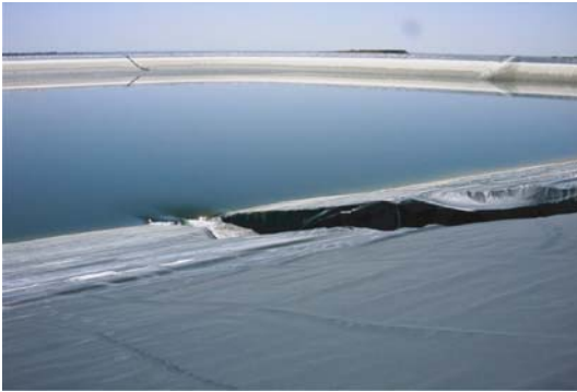
Fig. 11 Upstream view of dam after failure
