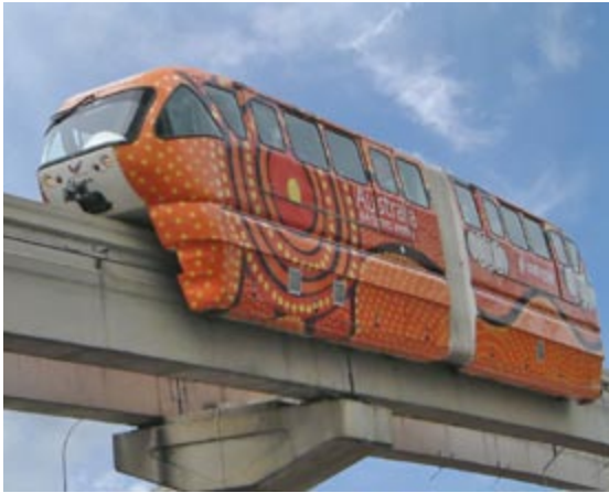
Fig. 2.49 A pedestrian was seriously injured when a part fell from the Kuala Lumpur monorail during its initial trials. Photo by Calvin Teo
