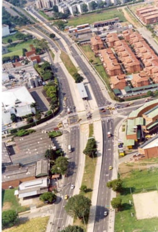
Fig. 20.7 and 20.8 The Cali (Colombia) system is an example of infrastructure development being far ahead of the business model. Without a business model in place, no vehicles can be purchased by the operators, and thus, the costly infrastructure is going unused.
