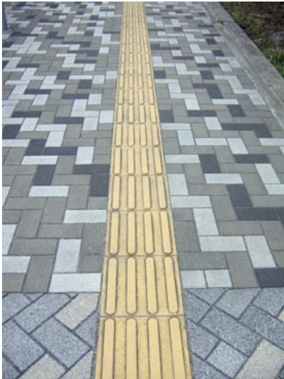
Fig. 13.82 Raised pavement markings can be a cost-effective way of providing safe access to the sight impaired.
