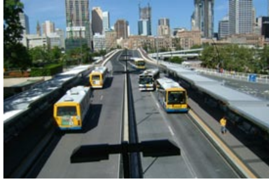
Fig. 3.20 and 3.21 Brisbane miscalculated demand at a major station resulting in significant busway congestion (left photo). The problem eventually had to be corrected through a somewhat costly retrofit of a passing lane at the station (right photo).
