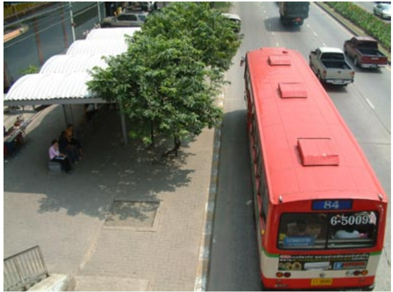
▲ Fig. 5.50 Curbside bus lanes are quite common in conventional bus systems, but often fail due to traffic congestion and poor enforcement.
