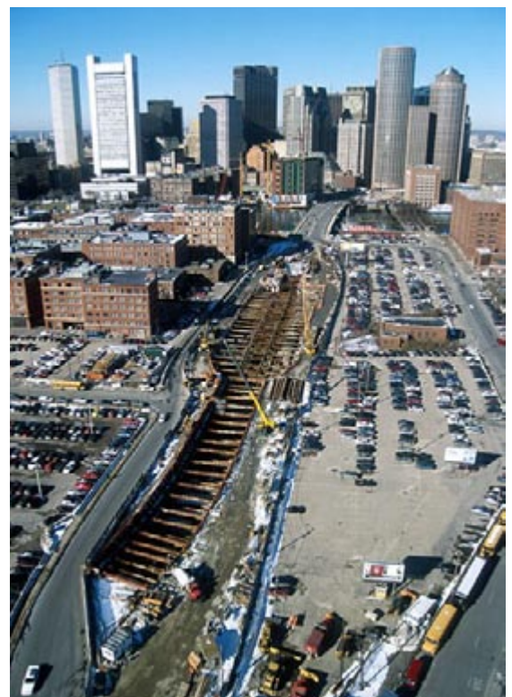
Fig. 5.29 The “Big Dig” in Boston included priority infrastructure for BRT.
