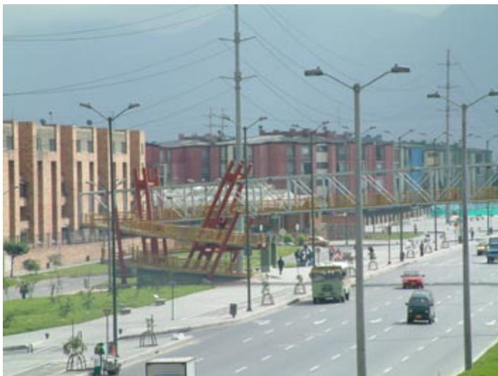
Fig. 13.48 In conditions where the BRT station is in the median of a multi-lane expressway, Bogotá utilises a pedestrian overpass.
