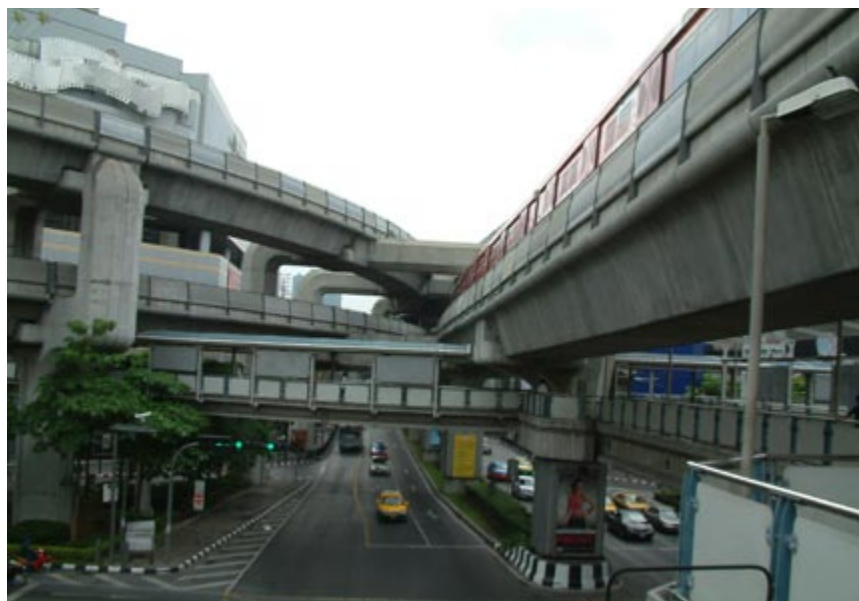
Fig. 2.59 The pillars supporting elevated systems, as shown here with the Bangkok Skytrain, can also consume a considerable amount of surface space, especially in the median and sometimes along footpaths.
