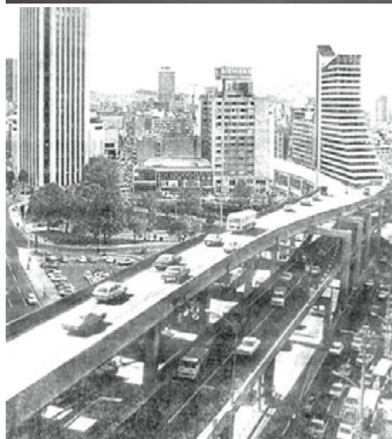
Fig. 3.12 A JICA drawing showing a vision for Bogotá with elevated roadways. Fortunately, Mayor Enrique Peñalosa rejected this vision and opted to build TransMilenio instead of elevated roads.
