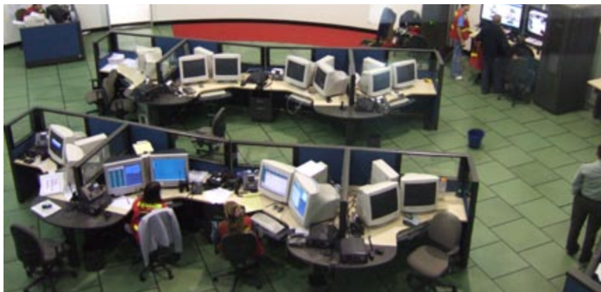
Fig. 11.123 The control centre should be designed with sufficient space for future expansion. Photo by Lloyd Wright
