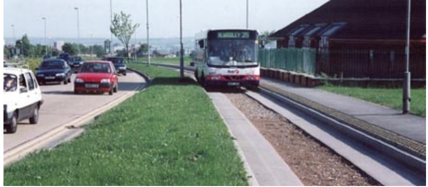
Fig. 11.25 and 11.26 Not paving the centre of the busway can produce infrastructure cost savings as well as reduce operational noise.
