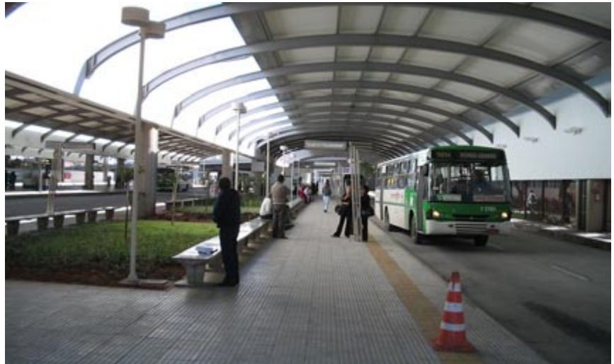
Fig. 10.27 The cleanliness of this terminal in São Paulo sends a positive message to customers. Photo by Dario Hidalgo
