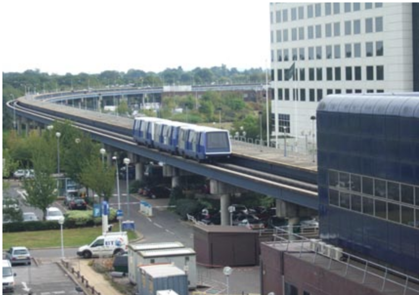
Fig. 15 A rubber-tyred vehicle on an elevated track provides public transport services between the terminals of London Gatwick Airport.
