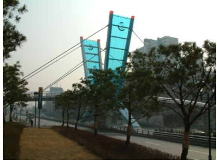
Fig. 13.54 The modernistic design of this pedestrian overpass in Seoul makes for a captivating sight.
