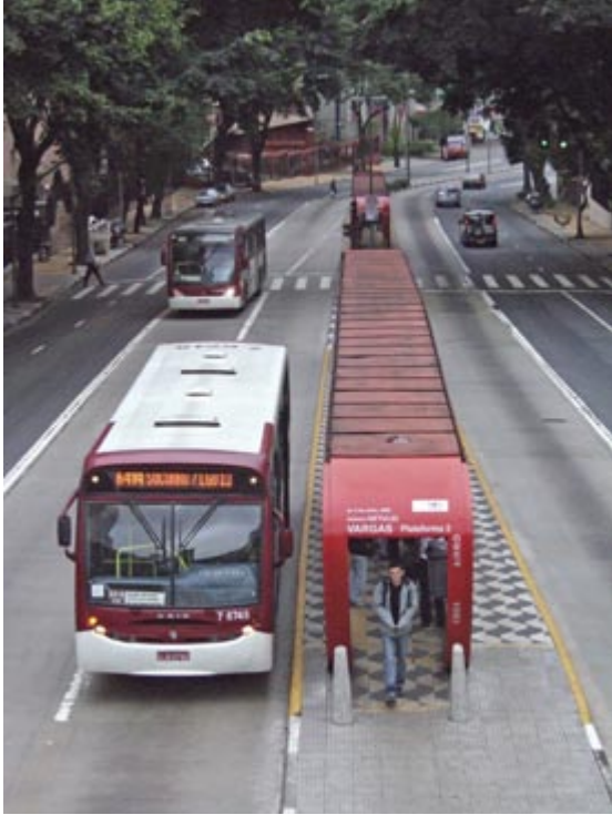
Fig. 4.8 São Paulo’s busways provide dedicated right-of-way to public transport outside the city centre, but once in the CBD most public transport vehicles no longer serve the area with priority treatment.
