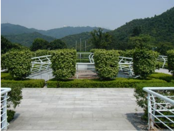
Fig. 13.53 A park-like environment makes this pedestrian overpass in Guangzhou (China) more inviting.
