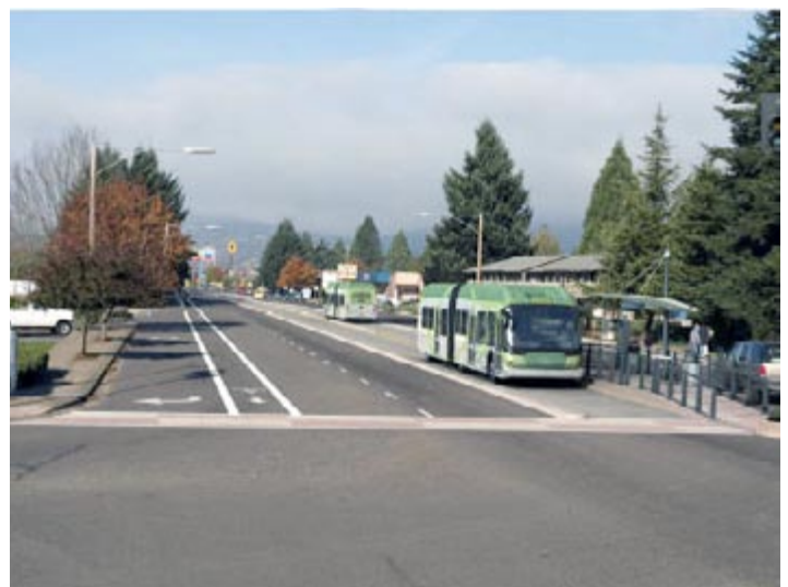
Figure 5.64 Vehicles with doorways on both sides permits Eugene to share a single lane for both directions at a station.
