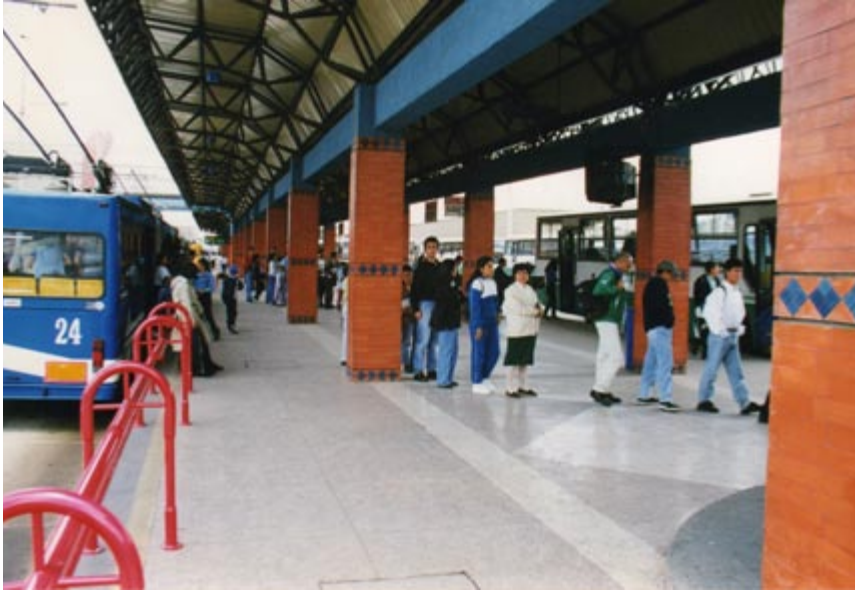
Fig. 11.93 At the El Recreo terminal of the Quito Trolé, customers easily transfer from trunk services to feeder services by crossing a platform. Photo by Lloyd Wright
