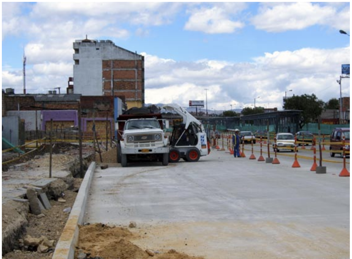
Fig. 11.133 Land and property expropriation in Phase II of TransMilenio greatly increased the overall capital investment.
