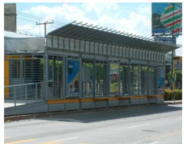
Fig. 11.59 While this roof overhang in León provides shading to passengers along the platform, many consider it to be aesthetically unappealing.
