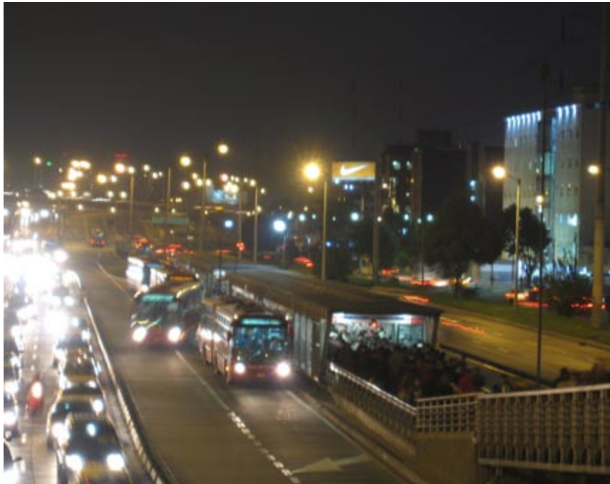
Fig. 2.41 The provision of multiple stopping bays and passing lanes at stations permits the Bogotá TransMilenio system to achieve high passenger capacity.
