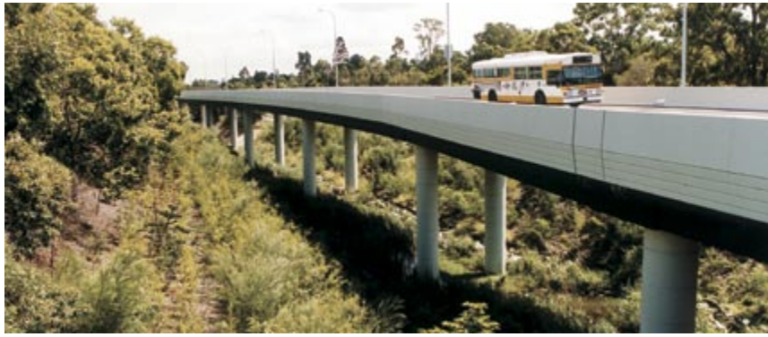
Fig. 11.29 An elevated busway in Brisbane allows the system to manoeuvre through a sensitive greenway.
