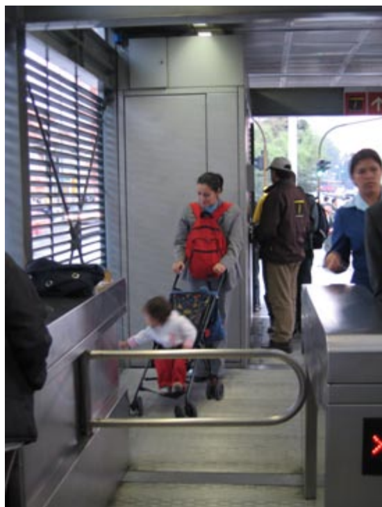
Fig. 12.67 A drop-arm turnstile option is provided for customers with special needs in many TransMilenio stations. Photo by Carlos F. Pardo
