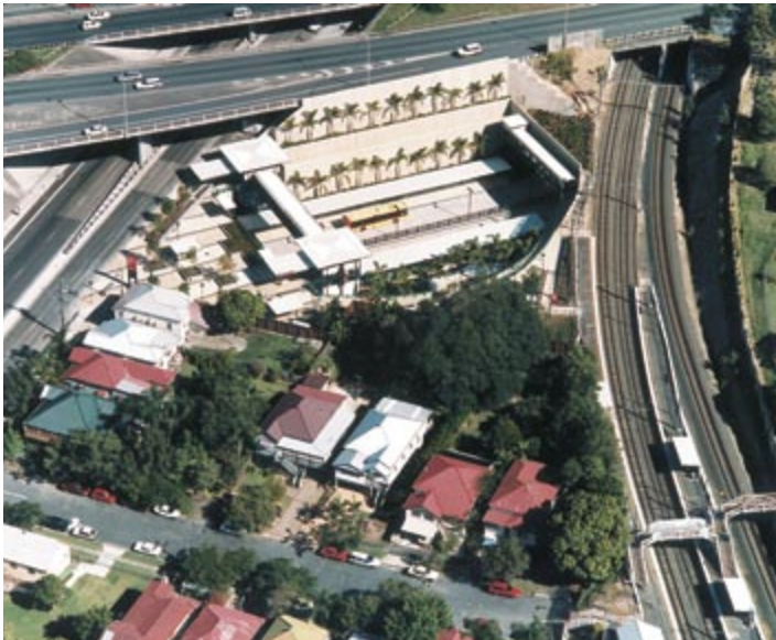
Fig. 13.108 The Brisbane Busway (top centre) is closely integrated with the city’s commuter rail service (right).
