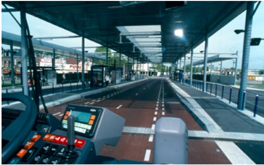
Fig. 30 The BRT systems in Rouen (photo above) and other cities of France have introduced many new features, especially high-technology vehicles and guidance systems. Image courtesy of Connex
