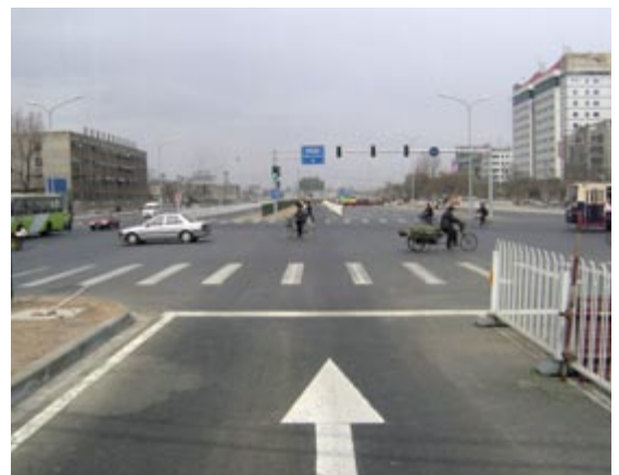
Fig. 3.26 The five-metre wide corridor in Beijing was quite wide for a single lane busway but insufficient for two lane operation.
