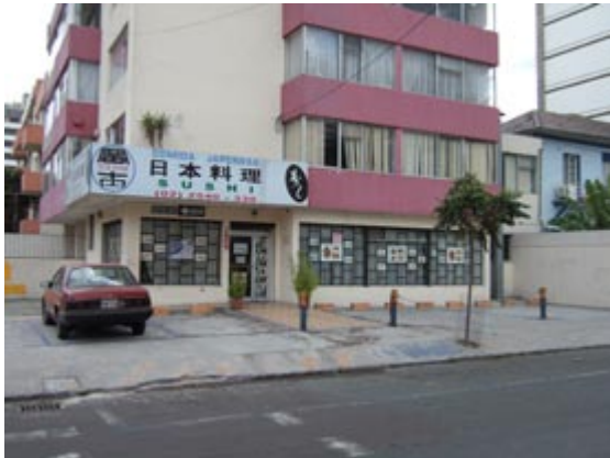
Fig. 14.5 With a parking space levy, shops have an inherent incentive to only provide the number of parking spaces that are truly required. Photo by Lloyd Wright
