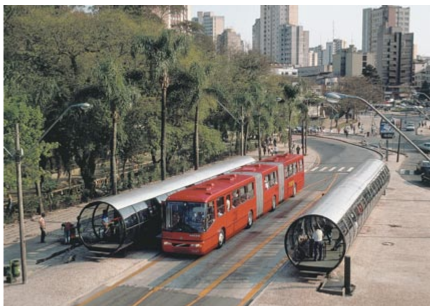
Fig. 8.15 Curitiba's innovations with station design and the station-to-vehicle interface did much to make BRT a high-capacity option. Photo courtesy of Volvo
