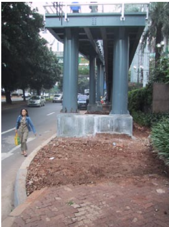
Fig. 13.5 Pedestrian Infrastructure of the new BRT System in Jakarta.
