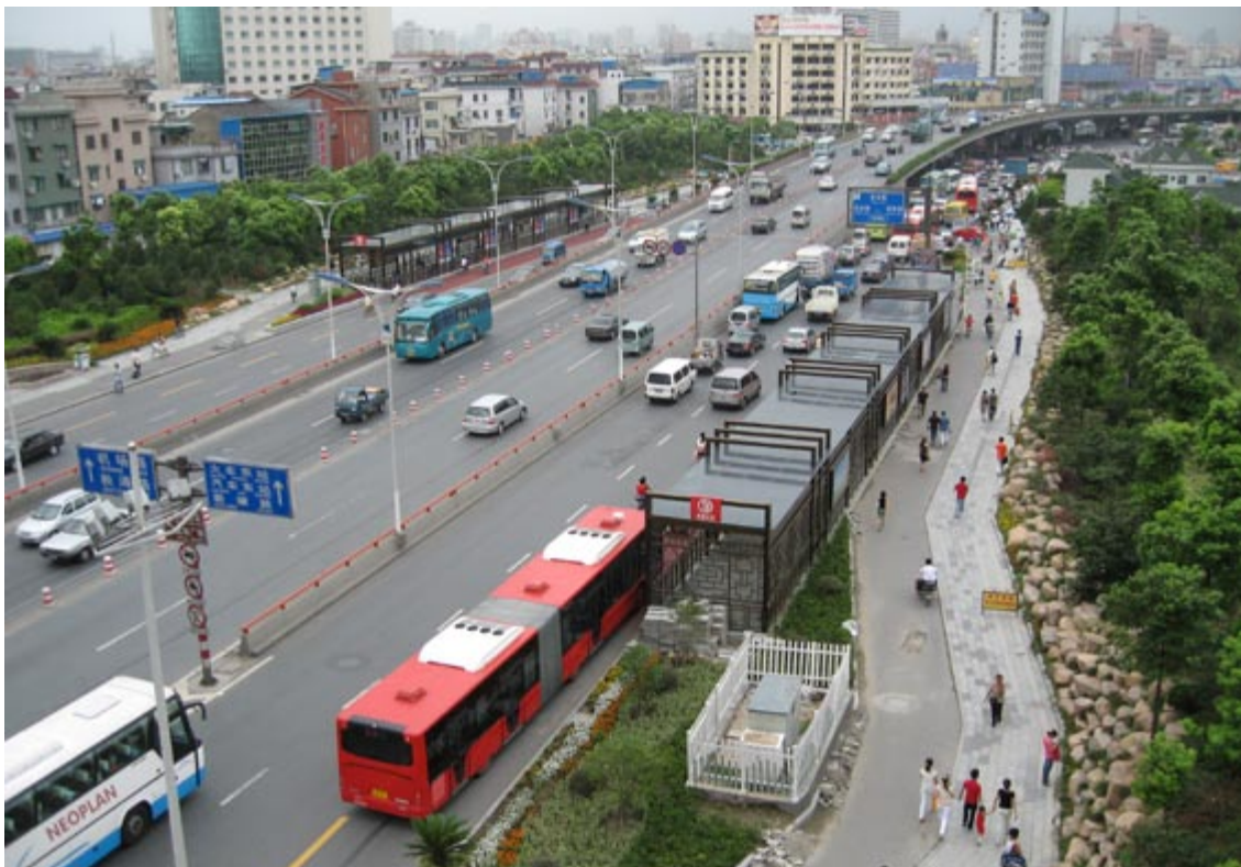
Fig. 13.102 The cycleway along the Hangzhou BRT system is sited between the BRT lane and the pedestrian footpath.
