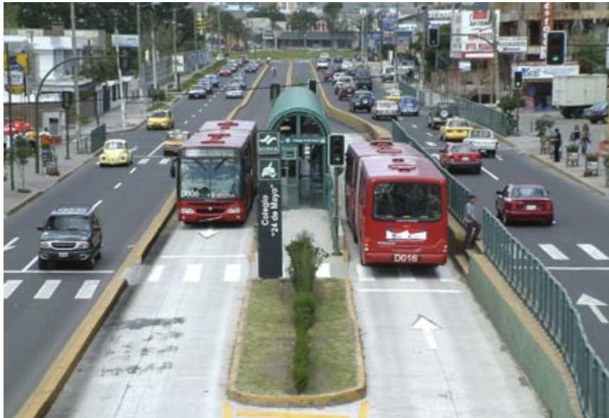
Fig. 5.6 The Ecovía corridor in Quito provides an example of a standard BRT road configuration. Photo by Lloyd Wright
