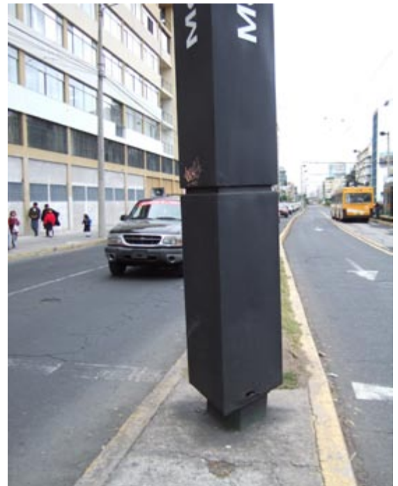
Fig. 13.61 This BRT identification post in Quito is placed in a pedestrian island, and acts to block the pedestrian’s view of both oncoming mixed traffic as well as oncoming BRT vehicles.
