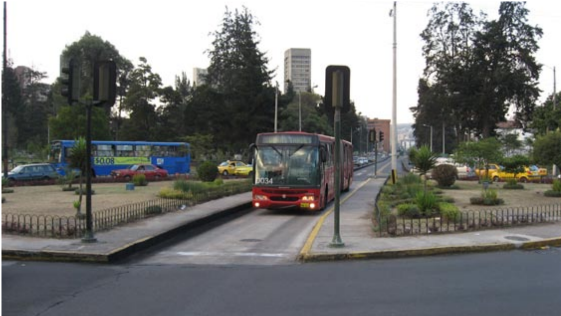
Fig. 9.52 Quito's Ecovía line cuts directly through a roundabout.
