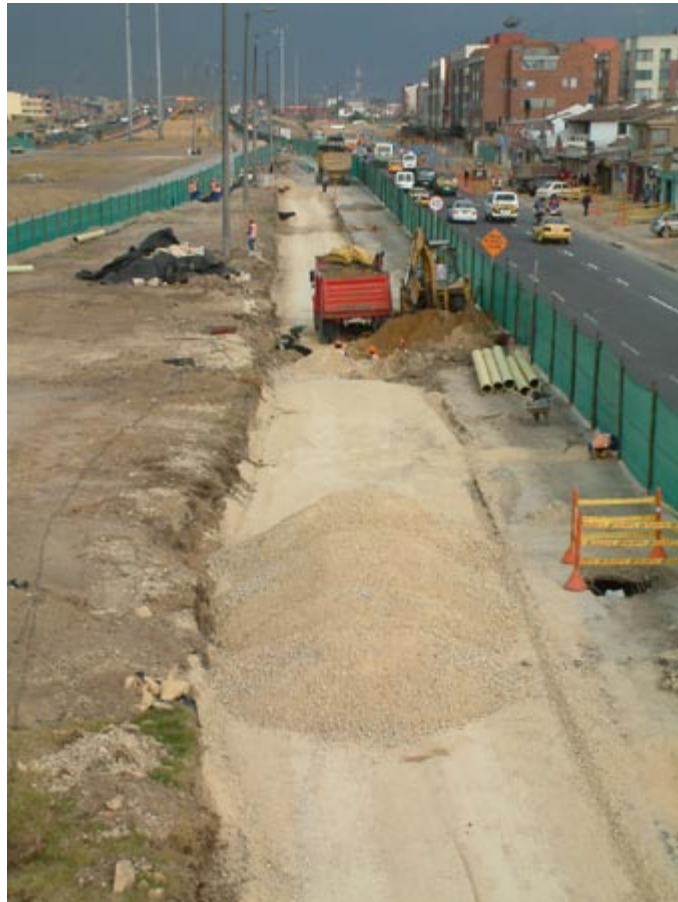
Fig. 20.29 Construction on the Americas corridor in Bogotá.
