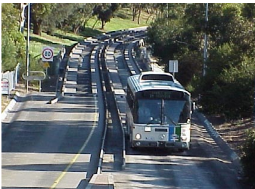
Fig. 11.24 Mechanically guided systems allow greater vehicle velocities and narrower busway width, but these systems to increase construction costs and reduce overall system flexibility.
