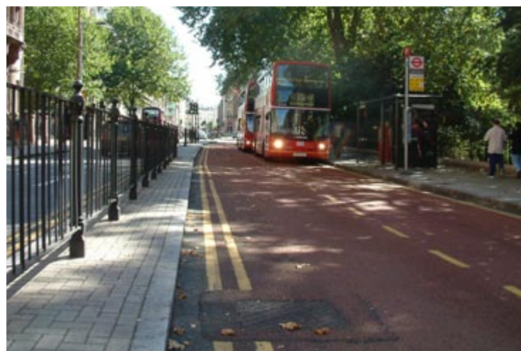
Fig. 11.129 Providing standard feeder vehicles with dedicated right-of-way at key junctures can do much to improve average travel speeds.
