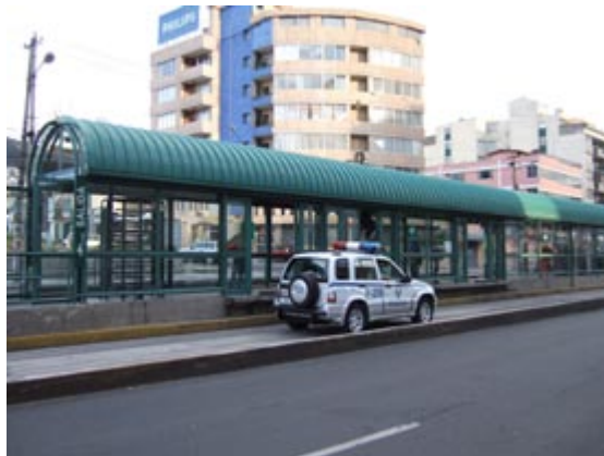
Fig. 7.1 and 7.2 In cities such as Quito, the exclusive busways also permit emergency vehicles to avoid traffic delays and respond more quickly to those in need. Photos by Lloyd Wright
