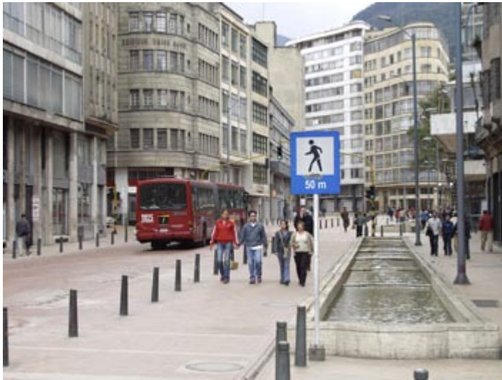
Fig. 13.32 Alameda Jimenez in Bogotá only allows BRT and non-motorised access.
