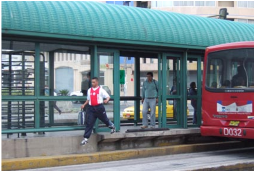
Fig. 11.60 Without sliding doorways, customers may evade fare payment and endanger their safety by entering and exiting through the platform doorway.
