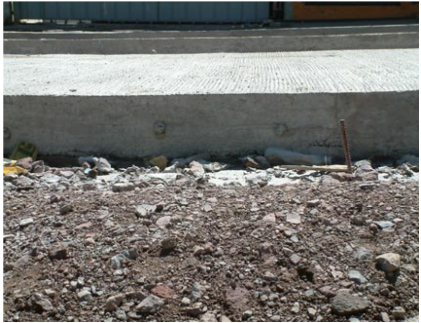
Fig. 11.6 Reinforced concrete, as in this example from the construction of the Quito Central Norte line, has much greater longevity than asphalt.
