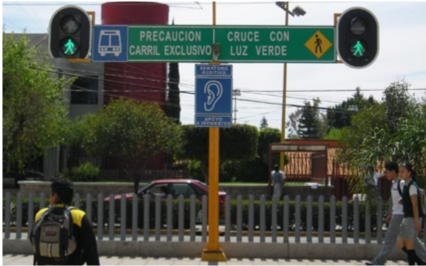
Fig. 13.84 Audible signal at a crossing leading to a BRT station in León (Mexico).
