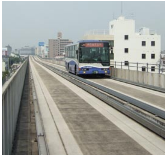
Fig. 5.30 The Yurikamome line in Nagoya utilises an elevated roadway structure to avoid any conflicts with street level traffic.
