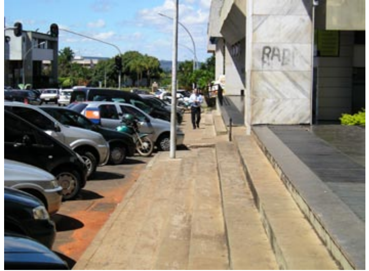
Fig. 13.66 These steps in Brasilia (Brazil) reduce the effective width of the footpath to less than 0.5 metres. Photo by Michael King
