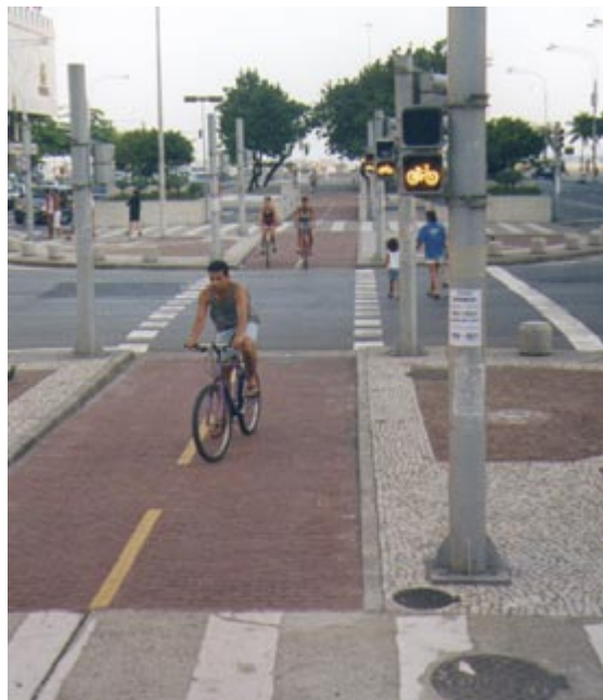
Fig. 9.26 A dedicated green phase for crossing cyclists is another effective solution as shown in this example from Rio de Janeiro.
