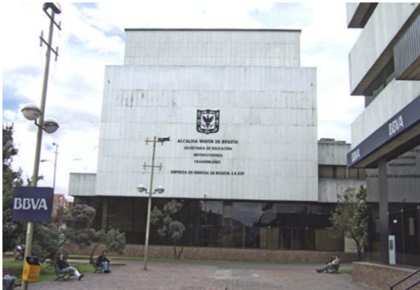
Fig. 3.2 Bogotá developed a new entity, TransMilenio SA, to oversee the development of the city's BRT system.
