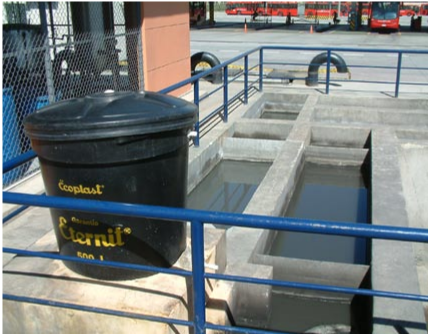
Fig. 19.28 A waste recycling facility at the Usme depot of TransMilenio. Photo by Lloyd Wright
