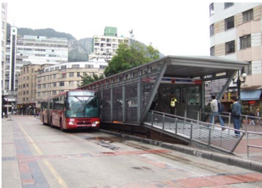
Fig. 20.28 The Eje Ambiental corridor in Bogotá. Photo by Lloyd Wright
