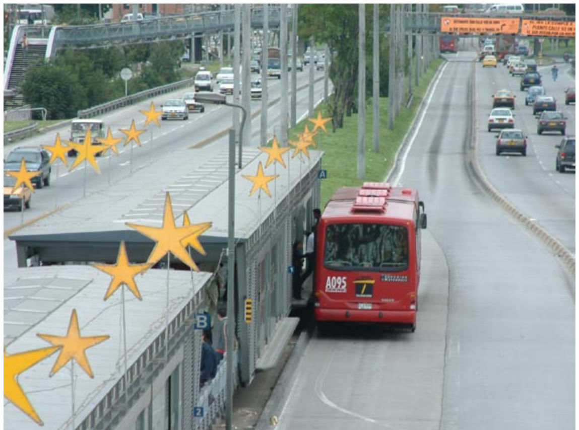
Fig. 11.41 At many stations within the Bogotá TransMilenio system, a transition area exists between a single lane busway and two lane configuration for passing.
