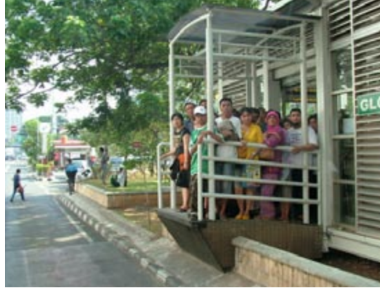
Fig. 8.31 and 8.32 The use of a single doorway in Jakarta has greatly limited the viable capacity of the system.
