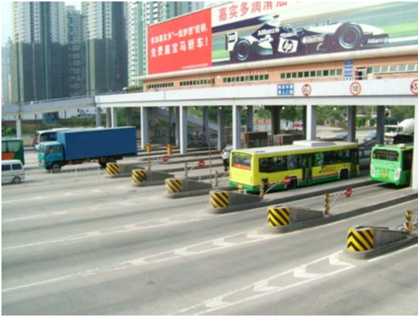
Fig. 13.35 Authors successfully testing an abandoned toll plaza on a high speed road in Guangzhou as a possible safe pedestrian crossing for a very wide high speed road.
