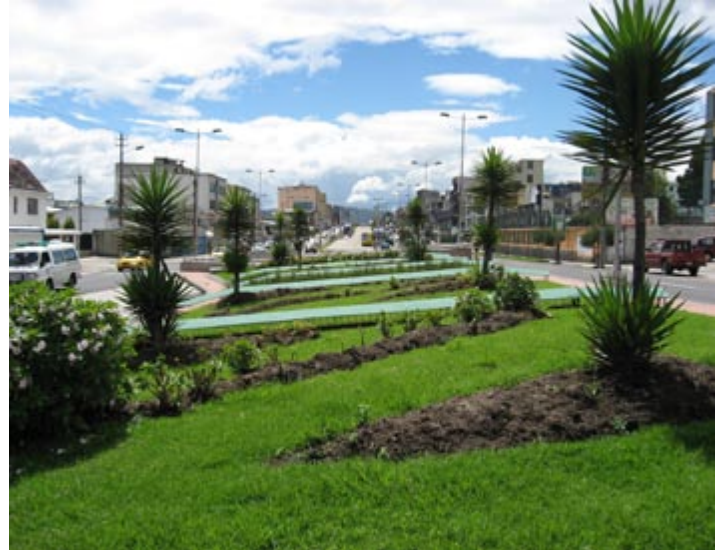
Fig. 11.39 The covering of a new BRT underpass creates new green space along the Central Norte corridor in Quito.
