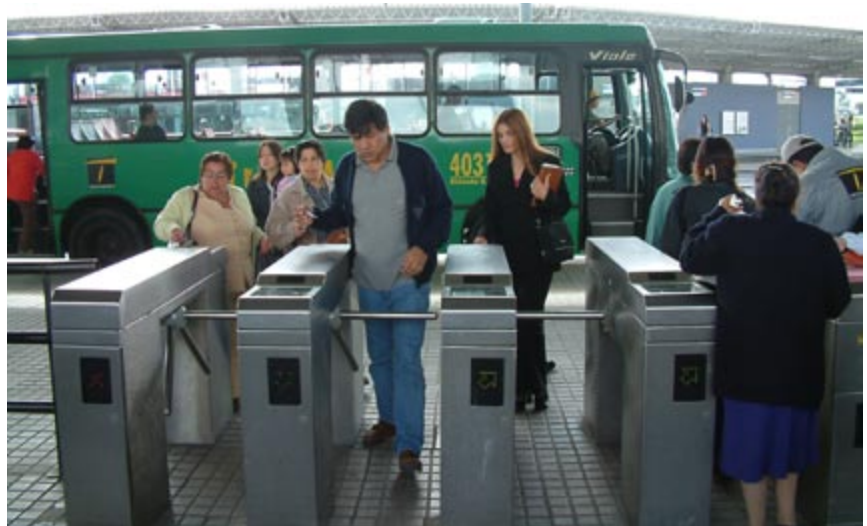
Fig. 12.65 Rotating-arm turnstiles, as utilised in Bogotá. Photo by Lloyd Wright
