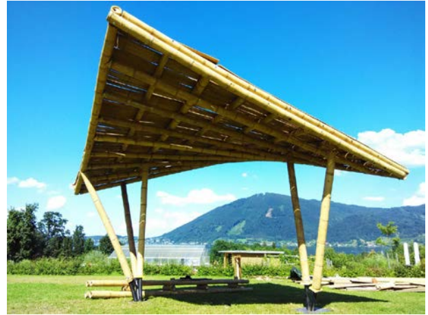
Figure 2: Prototype hypar constructed at the 2016 Base Habitat Summer School, Altmünster (Austria)
