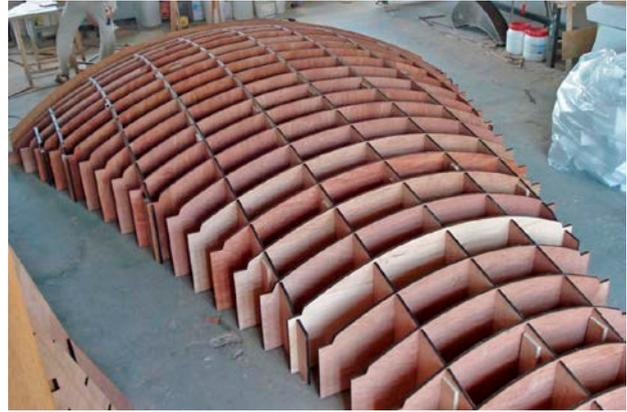
**Figure 9:** *Wooden rib system for the formwork [photo: Daniel Ehlig, TU Dresden], [29]*
