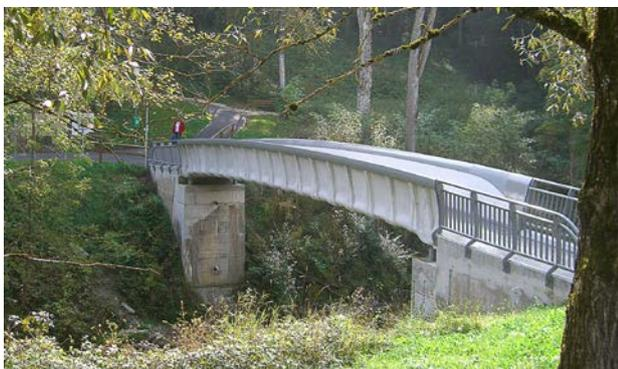
**Figure 7:** Textile reinforced bridge 'Rottachsteg' in Kempten [photo: Harald Michler, TU Dresden], [27]
