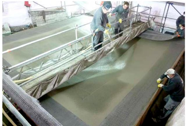
**Figure 13:** Manufacturing of the TRC hyperboloid shell layer by shotcrete [photo: © RWTH Aachen], [38]
