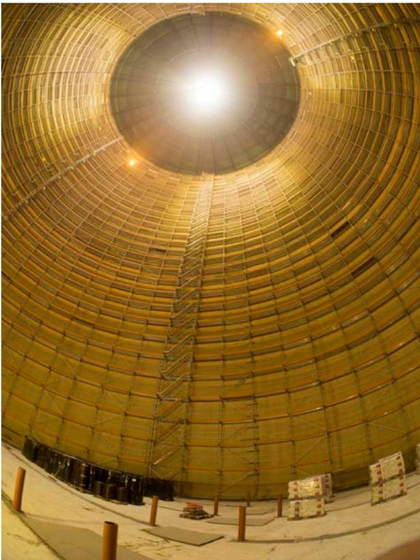
**Figure 21:** Scaffold inside of silo 9, Nordzucker AG Uelzen, during repair works with carbon reinforced concrete [photo: Harald Michler, TU Dresden], [49]
