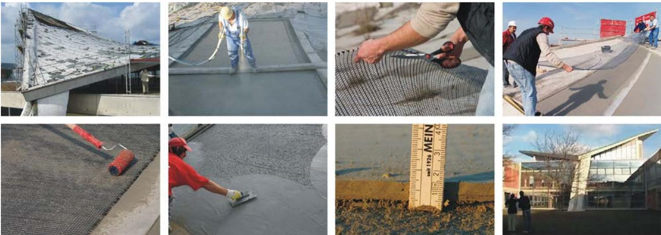
**Figure 20:** Strengthening of the hyper-shell in Schweinfurt (from top left to bottom right): before the measure, spraying of a first concrete layer, cutting, applying and slight impressing of a sheet of carbon reinforcement, smoothing the last concrete layer and checking of the layer thickness, ready strengthened structure [photos: Silvio Weiland and Ulrich van Stipriaan, TU Dresden], [48]
