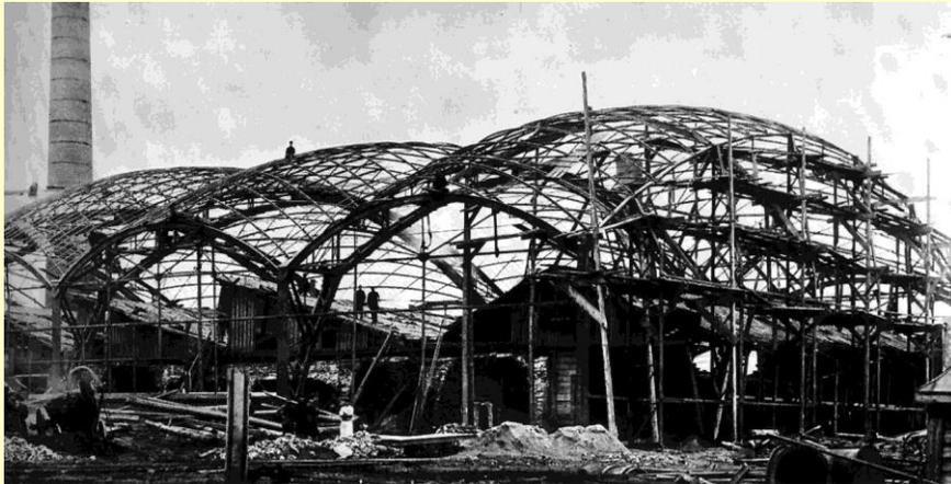
Description The double curvature diagonally framed Shell by Vladimir Shukhov in Vyksa near Nizhny Novgorod during construction, 1897
