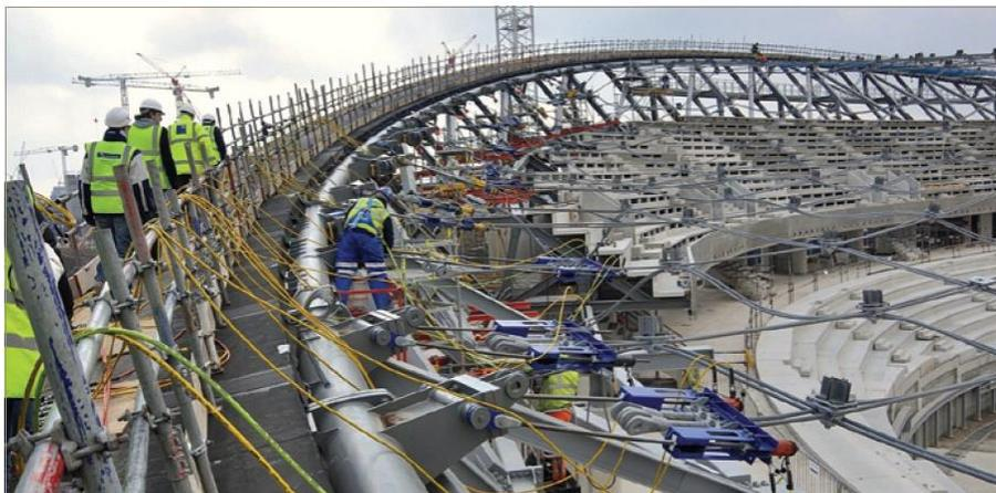
Figure 9. Cable net being jacked into position from the conveniently flat ring truss – installation forces in the 16 km of cabling were close to those predicted
