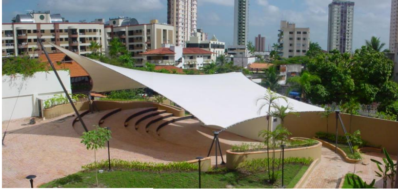
The membrane roof of the “Memorial dos Povos” of Belém do Pará
