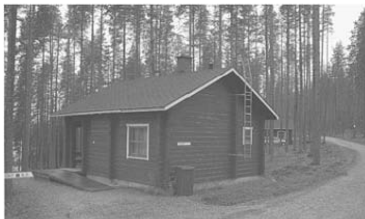
A well-designed traditional squared log cabin built to modern insulation standards. It is equipped for use by people with disabilities, and has an access ladder to the roof in case of fire. It is set amongst a pine forest of open character and stained a dull colour in order to fit in visually. Ruunaa National Hiking Area, Finland.
