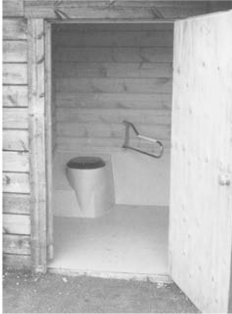
A view of a unisex disabled toilet cubicle with a wide door and movable handrail. The slight step into the building should be eradicated, as this will cause difficulties for wheelchair access.
