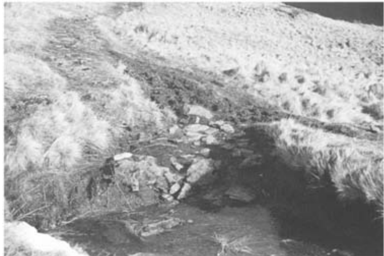
An example of an eroded path across peat. This is extremely difficult to restore or to lay a satisfactory path surface over. (Courtesy Peter Ford)
