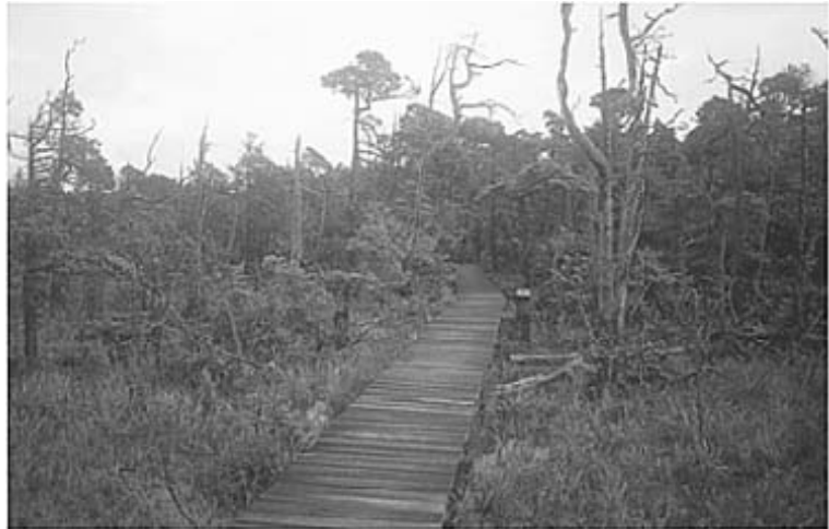
An excellent example of a floating boardwalk laid across bogland. The construction is of sawn timber resting on horizontal cross-bearers to spread the load. Pacific Rim National Park, British Columbia, Canada.
