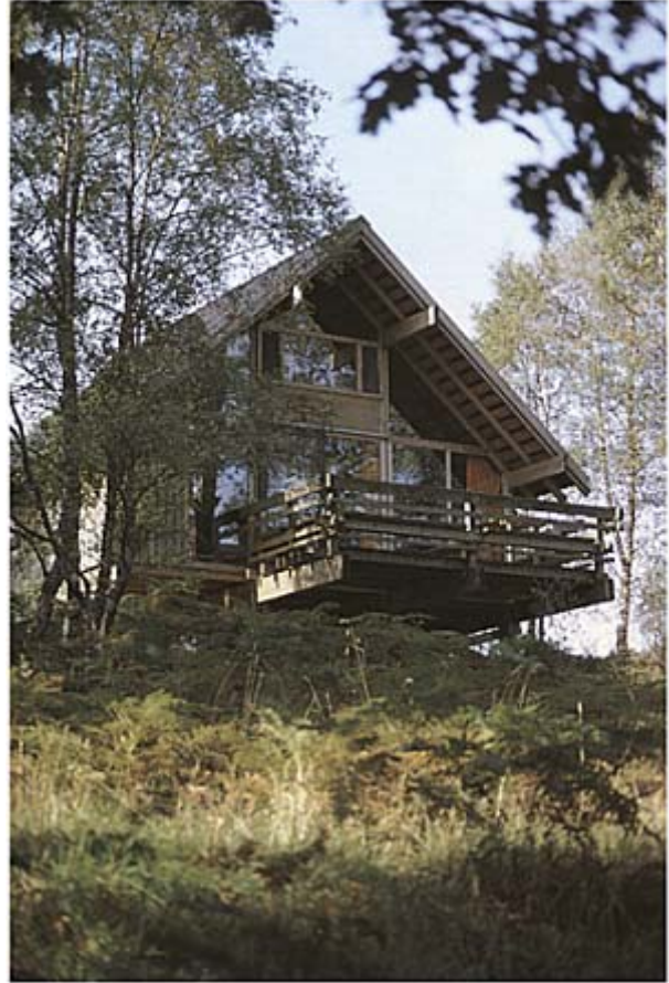
41 An attractive A-frame construction with large windows and a deck to give good light and a view over a lake. This example is supported on stilts to take advantage of a slope. Loch Awe side, Argyll, Scotland.
