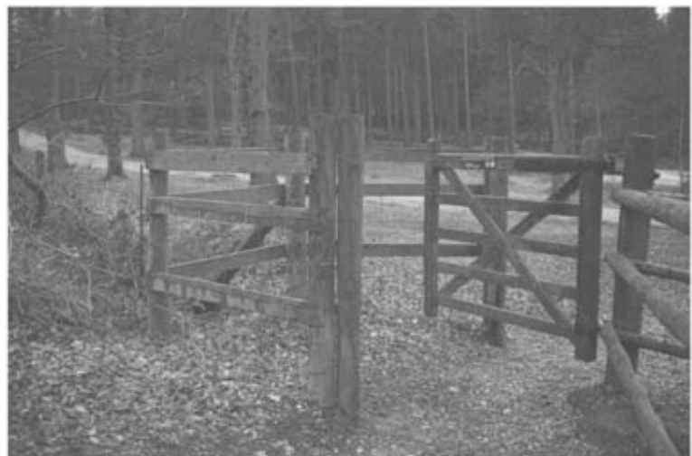
A kissing gate made so that wheelchairs or baby buggies can negotiate it. New forest, Hampshire, England.
