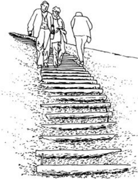
A 'sandladder' made from round timber crosspieces fixed to two steel cables. This permits loose, easily eroded material to be climbed safely and with a low risk of surface erosion. Mount St Helens, Washington, USA.
