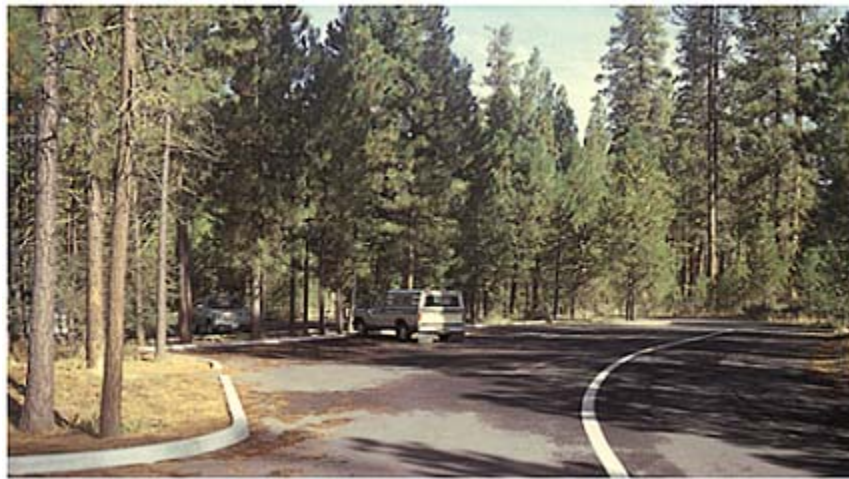
12 Forested car parks like this one help to provide shade for most of the day. This is important in sunny and hot summers, when cars can heat up severely if parked in the sun. The shade also reduces glare from surfacing. 'Head of the Metolius', Deschutes National Forest, Oregon, USA.
