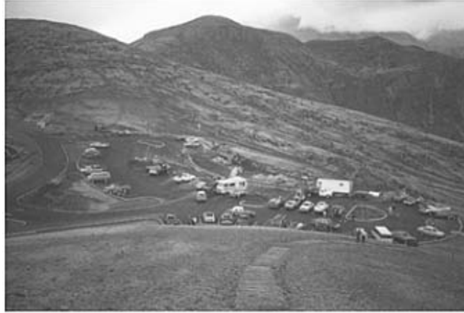
This area layout at Mount St Helens, Washington, USA, uses a natural bench in the landform to accommodate the parking. Small islands help to break up the parking and establish the vehicle circulation. Pullthrough bays are provided.
