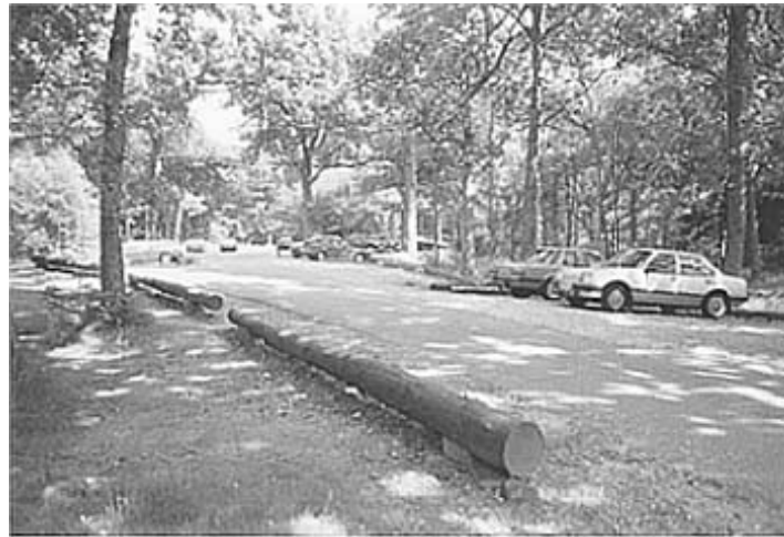
Horizontal log barriers of large size laid close to the ground are effective and fit into this wooded landscape of large trees.
