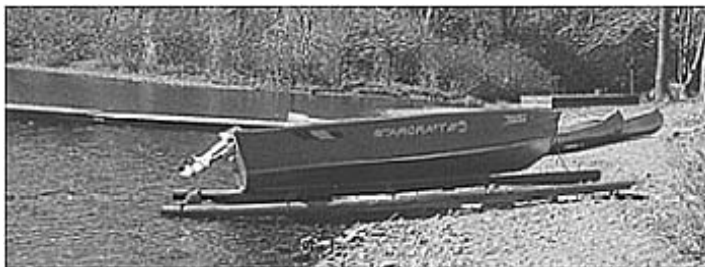
A simple, small boat-launching ramp, which uses rollers on a timber frame to ease the task of hauling a dinghy from the lake. Baxter State Park, Maine, USA.
