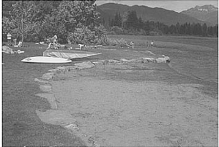
A lake beach where a low retaining wall has been laid in order to reduce the wear and tear of the grass edge along the beach. Whistler, British Columbia, Canada.
