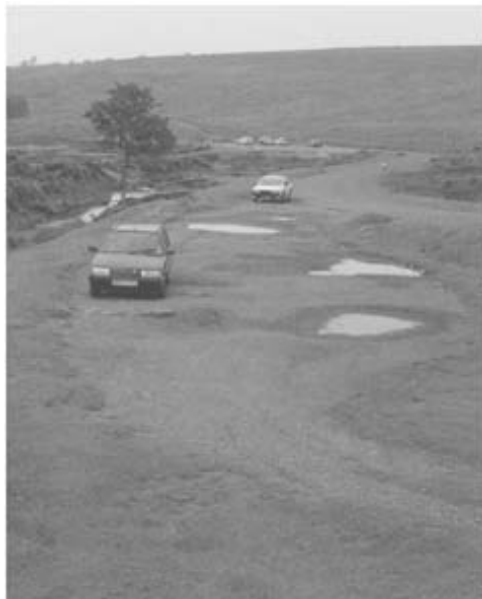
Unsealed surfaces can be subject to heavy wear and tear, erosion, potholing and puddles unless regularly maintained. 'Sheepwash', North York Moors National Park, England.
