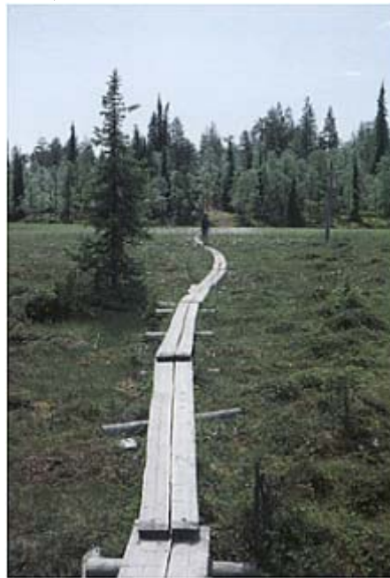
26 A boardwalk constructed of split logs cut from the nearby forest, borne on wide crosspieces to cross a mire in Finnish Lapland. All pieces are pegged together.
