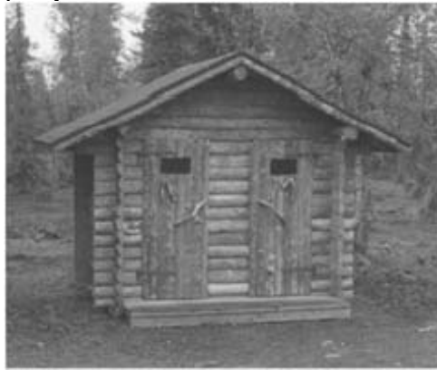
A toilet building made of logs at Akasamyly in Finnish Lapland. The result is a little 'rustic' because the logs are small. However, the main problem is the sole use of window holes cut into the doors to give light. This is inadequate, and may cause privacy problems.
