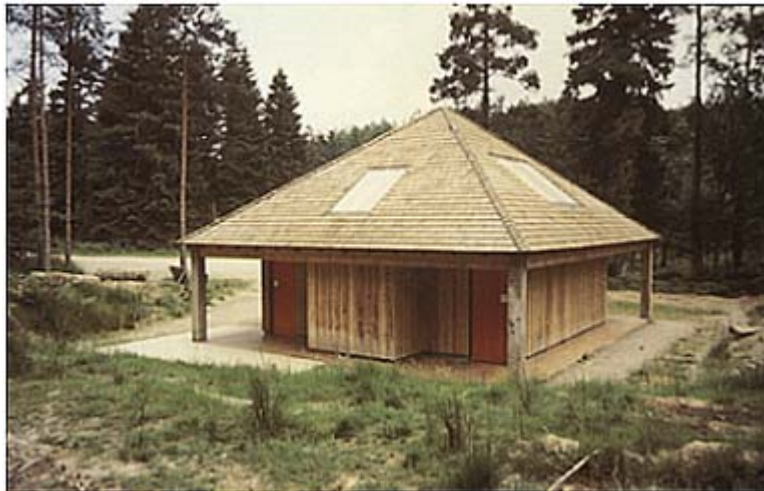
16 A large toilet building with over-hanging pyramidal roof of sawn timber construction. The large skylights give good illumination to the interior. Cannop Ponds, Forest of Dean, England.
