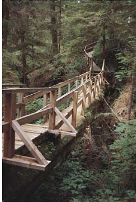
29 This bridge between two stretches of boardwalk has made use of a naturally fallen cedar log. The upper surface has been levelled, and a railing has been fixed directly to the log using coach screws. Pacific Rim National Park, British Columbia, Canada.
