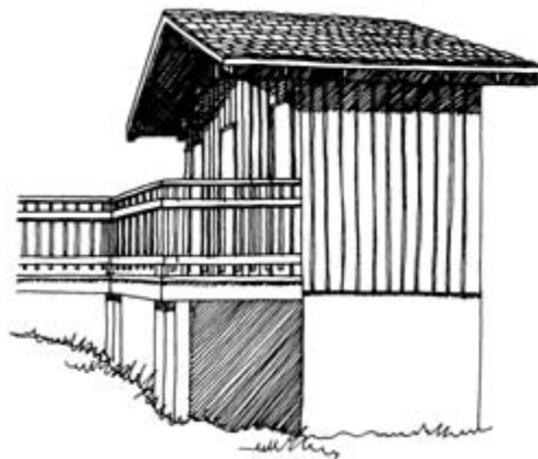
This toilet uses one of the proprietary composting systems such as the 'Phoenix' or 'Clivus Multrum'. The composting unit is built beneath the publicly accessible part of the building. The toilet is built on a side slope to avoid the need for stairs or ramps. This one is at a rest stop along Highway 1 on Vancouver Island, Canada.
