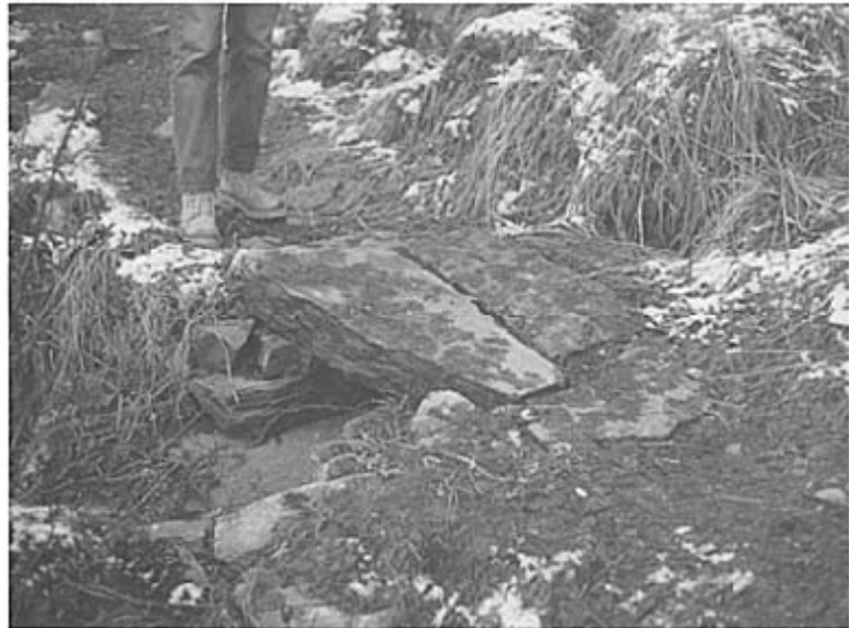
Culvert construction: (a) Modern culverts are easily made from lightweight plastic tubing laid in a trench cut to a fall across the path. (b) A stone culvert can be made from local materials. This is set beneath the path. (c) A plan view shows the layout of the culvert—its entrance contains a silt trap and its exit is dressed with stone. (d) A section through the culvert, showing the silt trap, the retained path edges and the culvert mouth set around with stone. (e) The culvert exit is tied into the path edge using stone to prevent erosion and to make a tidy result.
