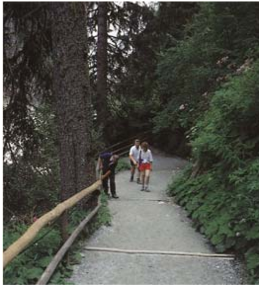
25 This wide, well-constructed path on a steep incline is well provided with cut-off drains or waterbars made from halfround logs with a channel cut into them. Krimml, Austria.
