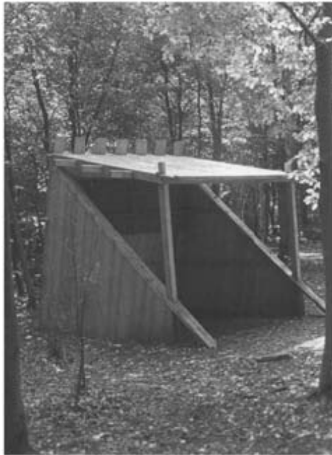
An interesting small shelter along a trail, made in four prefabricated sections, which are fitted together on site. This offers shelter or shade depending on the weather.
