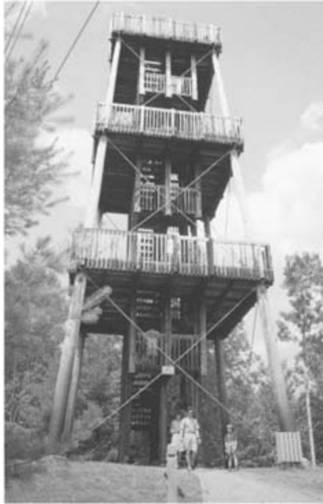
A viewing tower is an exciting feature, which elevates the viewer well above the tallest tree tops. Coaticook Gorge, Quebec, Canada.
