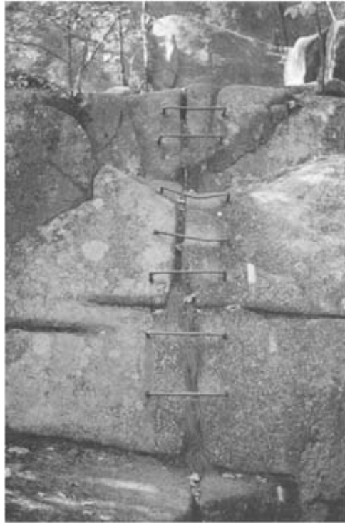
This set of steel steps is part of a formidable and challenging trail up a precipitous series of rock cliffs and ledges. They present a physical challenge only a little less than that of rock climbing, where ropes are needed. However, they are not particularly attractive. Acadia National Park, Maine, USA.
