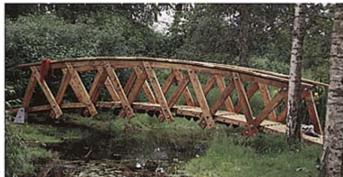
30 An arched bridge made from small sections of timber formed into a truss of great strength. Developed for Scottish National Heritage. (Courtesy David Downie)
