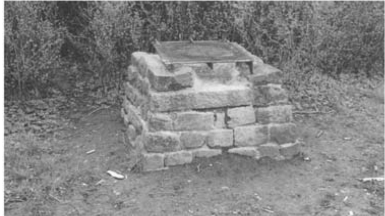
A stone-built altar fire with a hinged steel grill, which can be lifted out of the way. This is quite well built, but the surroundings are rather muddy. West Forest, Copenhagen, Denmark.
