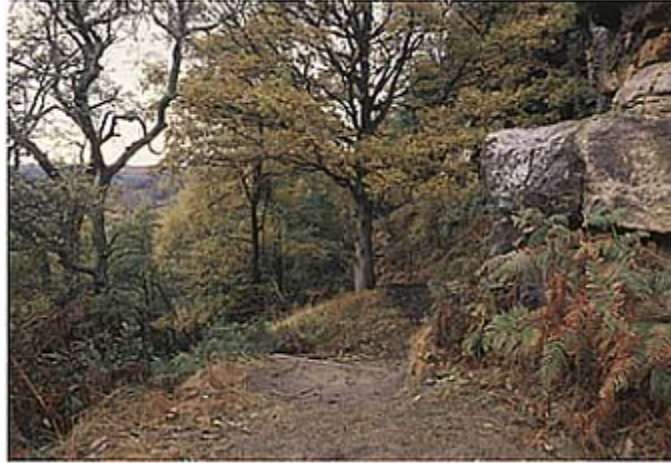
27 A good example of a path cut in a side slope on mineral soil. Re-vegetation of the slope and a good, well-drained surface result in the path's blending into the landscape very well.
