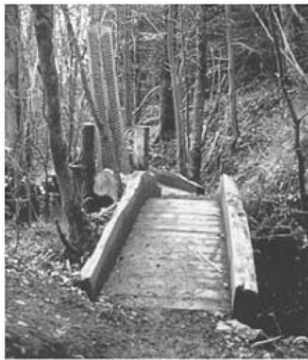
This interesting bridge has a drawbridge section on it. Walk on to it and it descends, allowing a person to cross. Haldon Forest, Devon, England.
