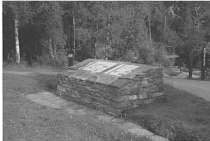
A stone structure used as the base for an information sign. Although used in a forest this might be more suitable in an open rocky landscape where stone is a dominant material. The workmanship of this example is good, but there is wear and tear around the unpaved sides of the structure. Glen Affric, Scotland.
