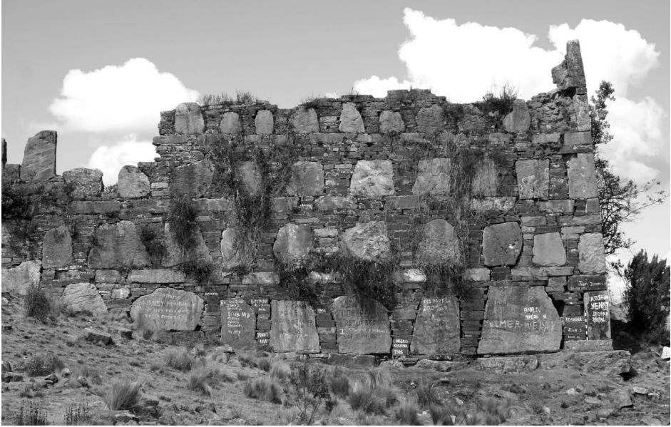
Figure 7. West façade of compound c40, Yayno (4,150 m above sea level). High-status buildings, such as this residential compound, feature strong inward batter, wanka-pachilla stonework, and rows of large stones of diminishing size. The wall surfaces are now targets for graffiti and vandals. The measure stick, lower right corner, is 1 m tall. © Photograph George F. Lau.
