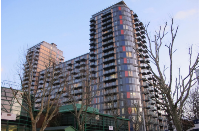
Figure 2.2.5 SOUTH boundary residential building
