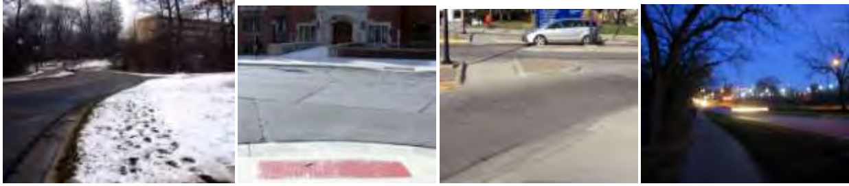
Figure 3-22 Basic pedestrian deficiencies on the U-M campus and adjoining streets include the absence of sidewalks, crosswalk striping, ADA-compliant curb ramps, and adequate lighting.
