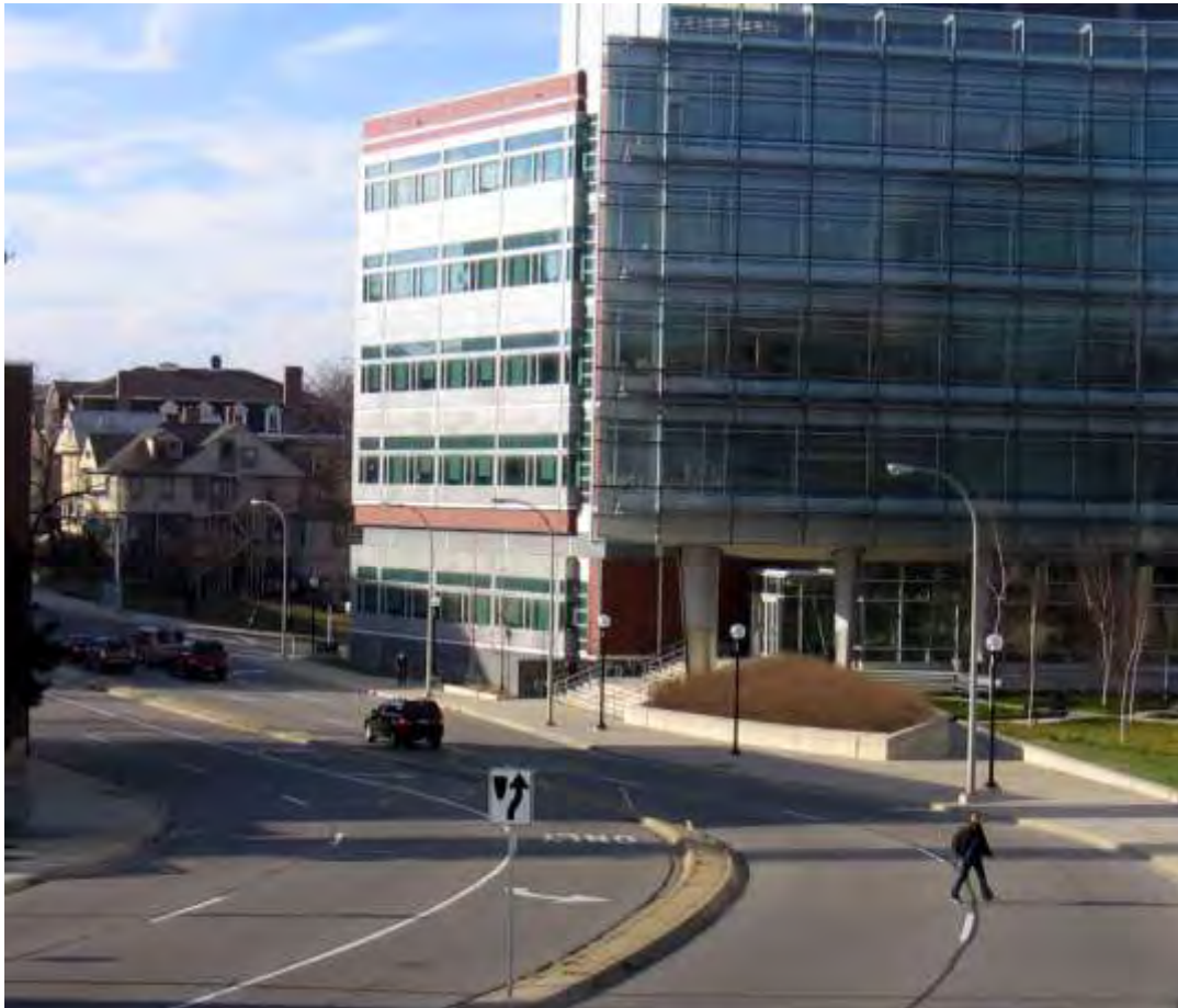
Figure 3-31 Pedestrian crossing Huron St. by U-M Bioscience Research Building.
