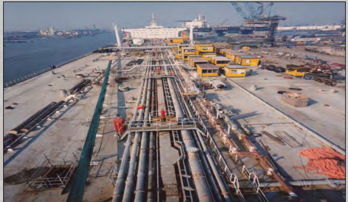
View from forward to aft while under construction in Rotterdam
