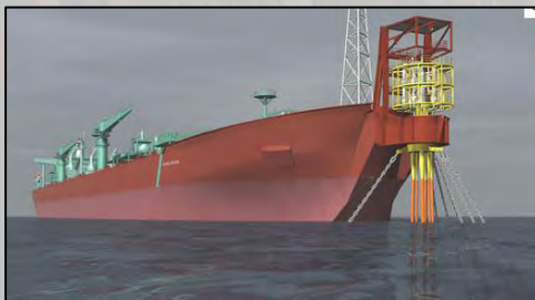
Single Point Mooring
