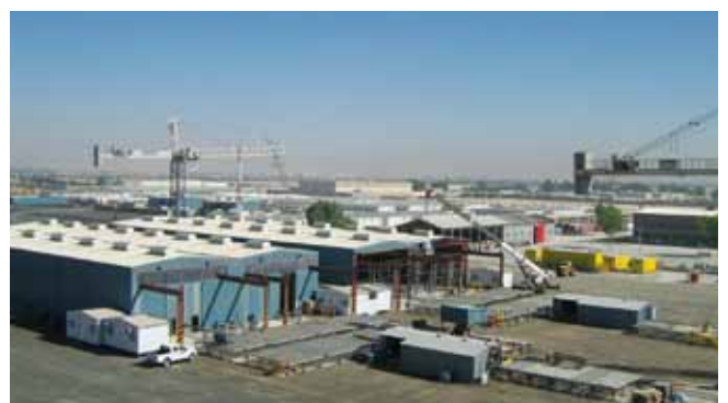
Dammam Onshore Fabrications Facilities, Dammam Saudi Arabia
