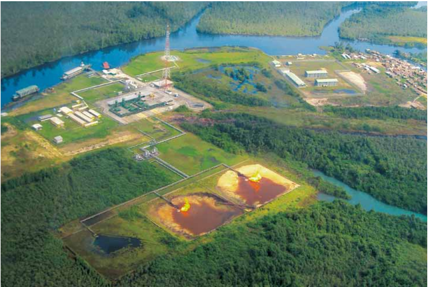
Project location with some initial site preparation.
