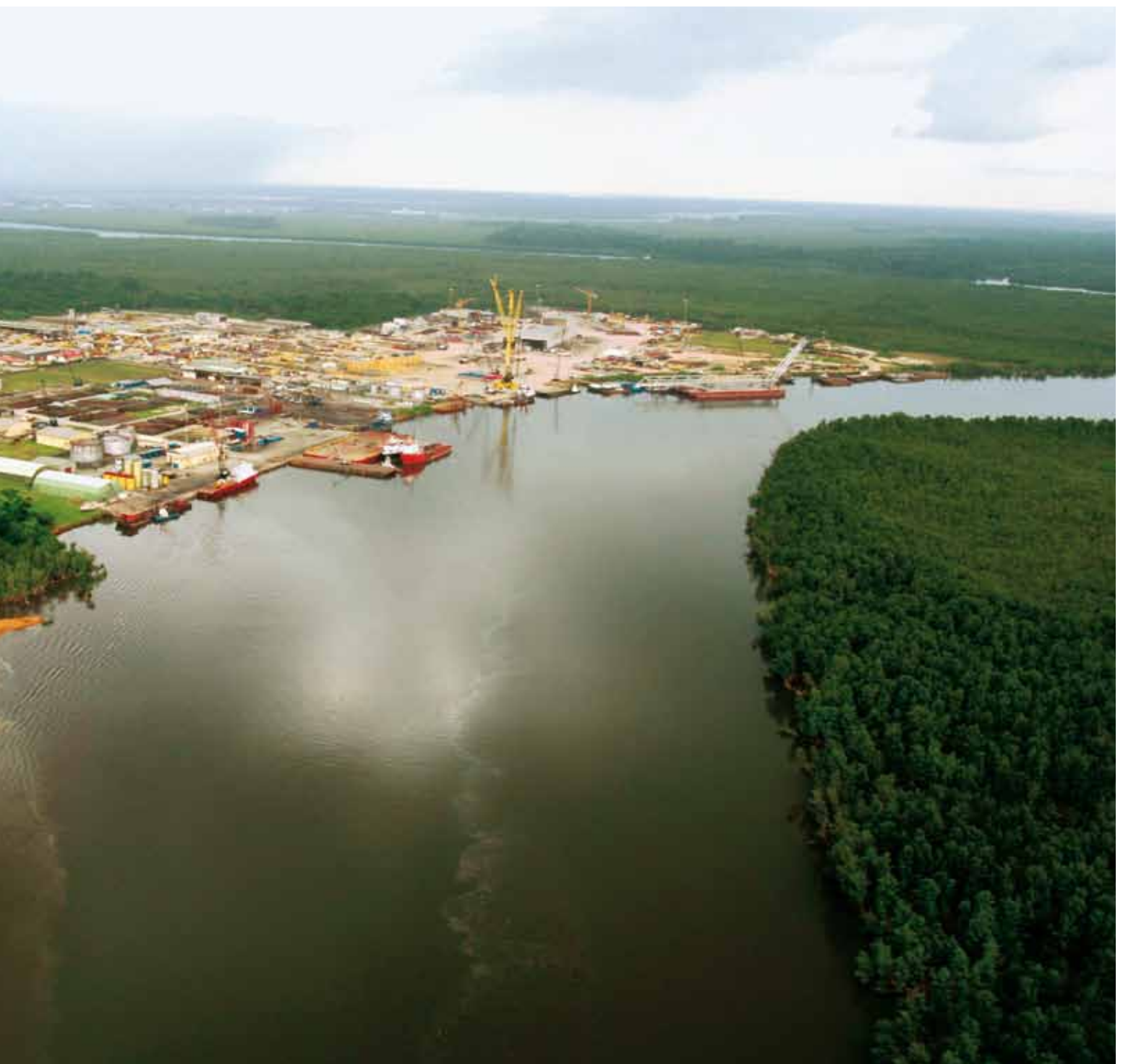
Saipem prefabrication and construction support yard at Port Harcourt - Rumuolumeni Base, Nigeria.
