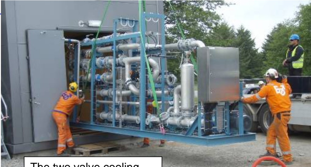
The two valve cooling skids lifted/slide in place
