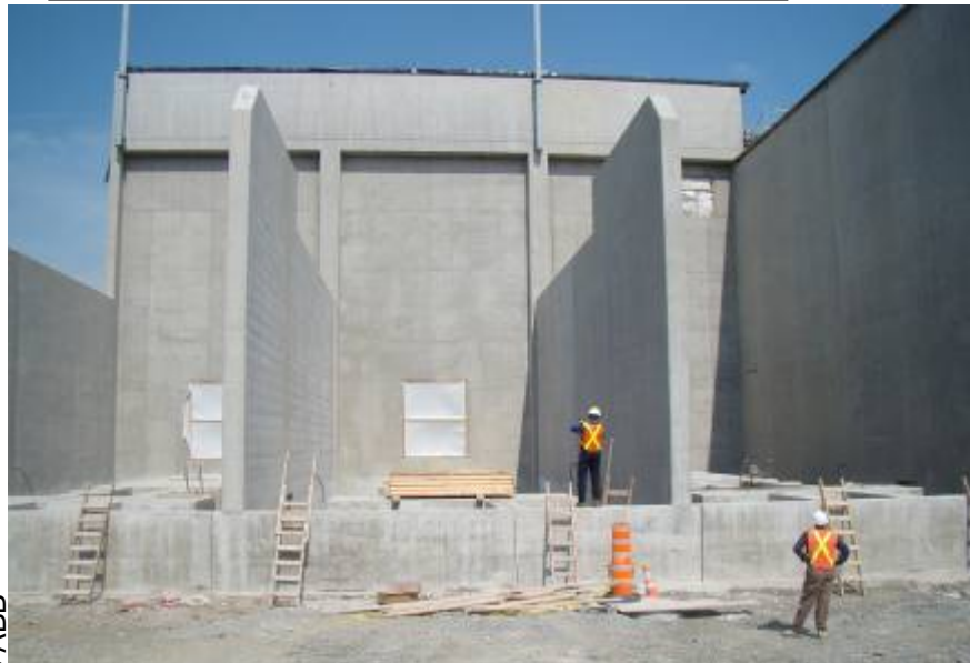
June, 10 – 240kV BI.01 trafo foundations
