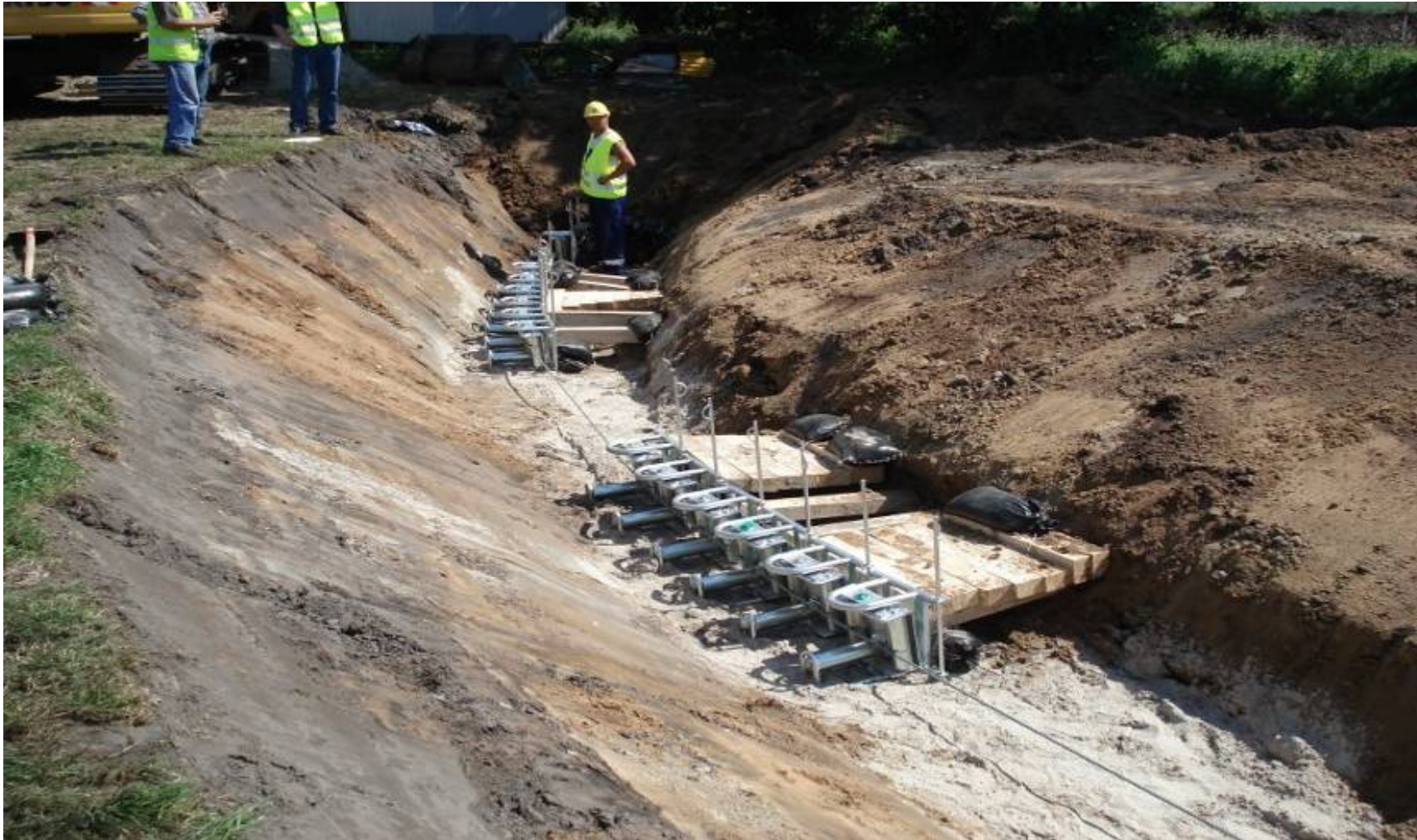
2008-06-09 First cable pull
