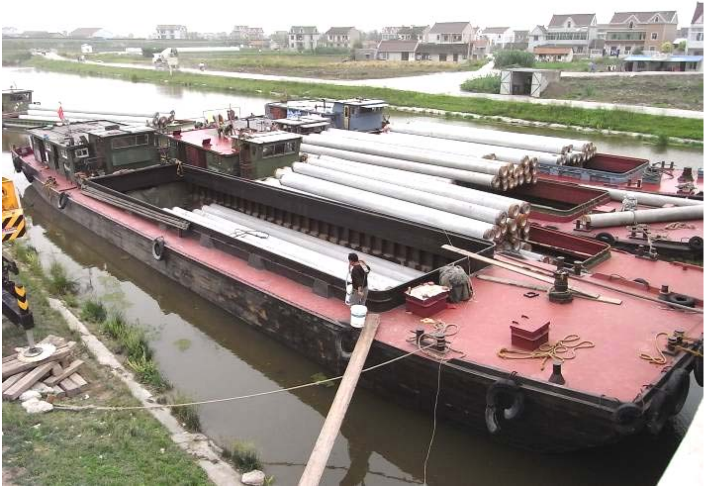
The piling material is transported to site in barges.
