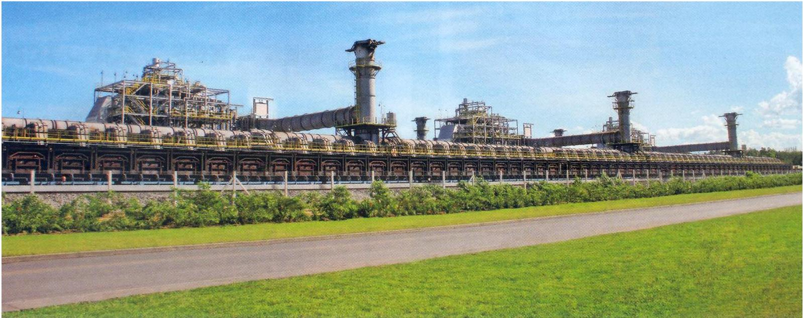
Coke oven battery with three heat-recovery boilers
