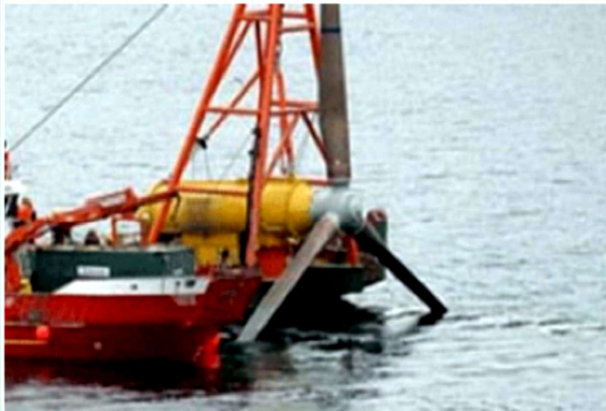
Deployment of the first grid connected marine turbine in Kvalsundet (Norway)
