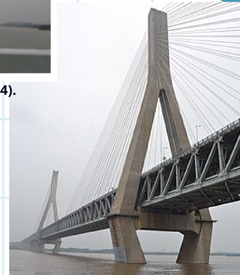
Qipanzhou Yangtze River Highway Bridge
