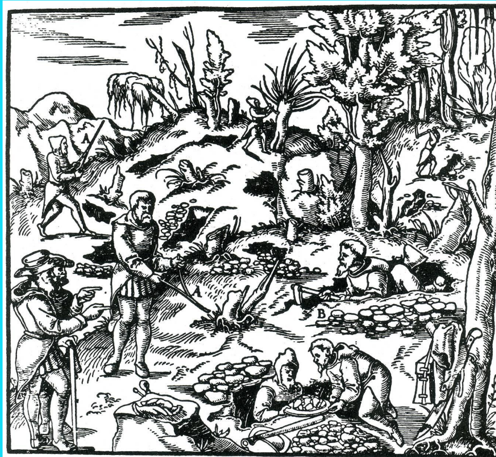
FIG. 1.3. Prospecting with a forked stick (A) and trenching (B) in the fifteenth century. (From Agricola, De Re Metallica , translated into English. Dover Publications, New York, 1950.)
