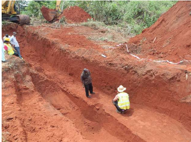
Fig. 4 Mechanical trench excavation of a moat at Benin
