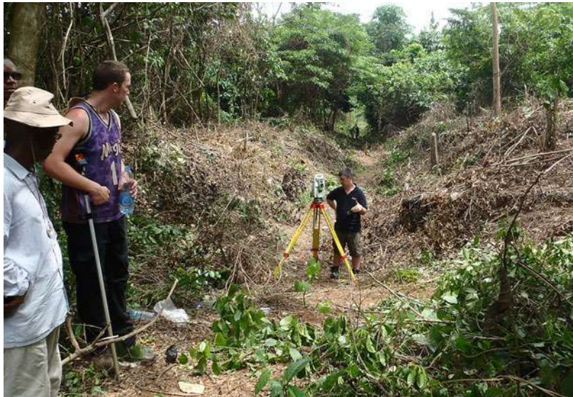
Fig. 2 Setting up Total Station for mapping in Benin
