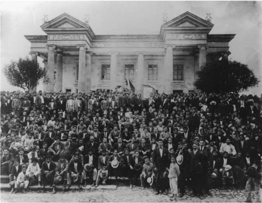
10. Inauguration of the new façade of Quetzaltenango's municipal theater built by Agatón Boj, 1907. Photograph by Tomás Zanotti, courtesy of CIRMA.
