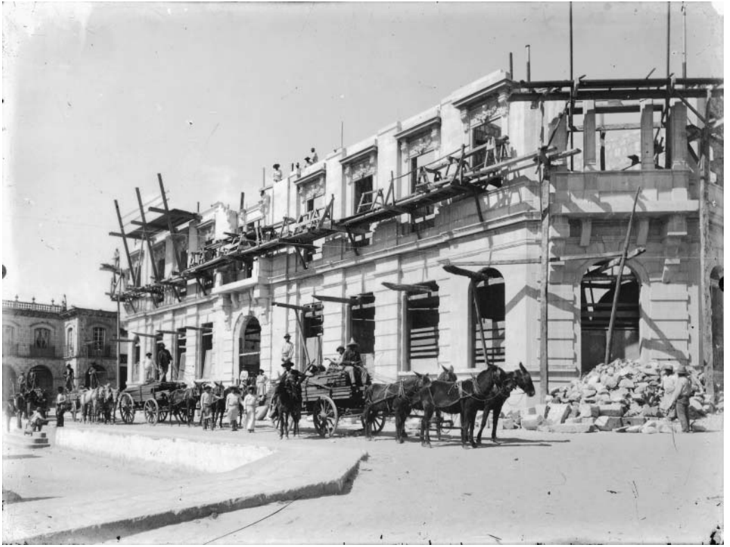
12. Building the second floor of the Banco de Occidente, c. 1910.
