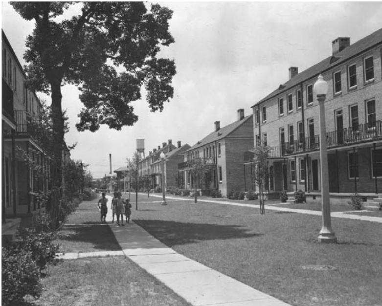
The Federal Housing Authority completely rebuilt St. Thomas Street in New Orleans, one of thousands such renovations. Here we see photos of the block before and after the U.S. Housing Authority came through in 1940. Courtesy of the Franklin D. Roosevelt Library Digital Archives.
