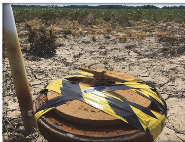
Figure 2. Sealing an alfalfa valve to prevent it from contributing additional irrigation water.
