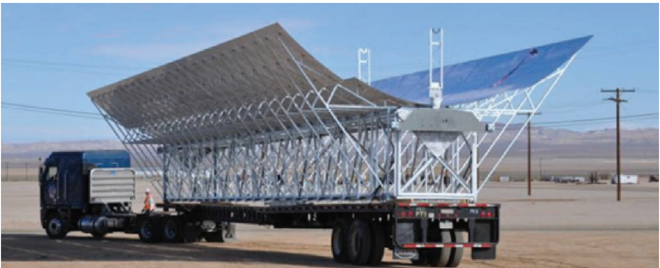
Figure 28: UltimateTrough collector during transport on site
