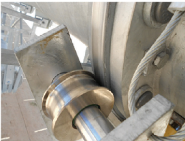
Figure 27: HelioTrough collector bearing at middle pylon [17]
