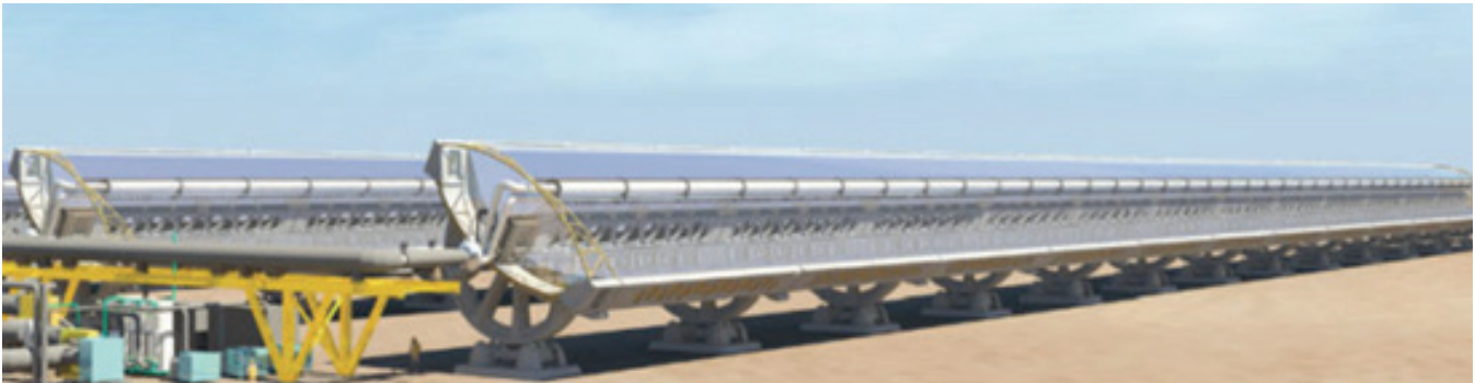
Figure 38: Parabolic trough collectors using concrete as main structural material [25]
