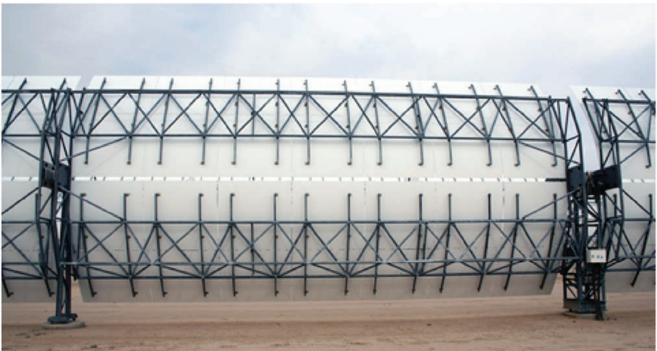
Figure 19: LUZ LS-3 collector from backside [12]
