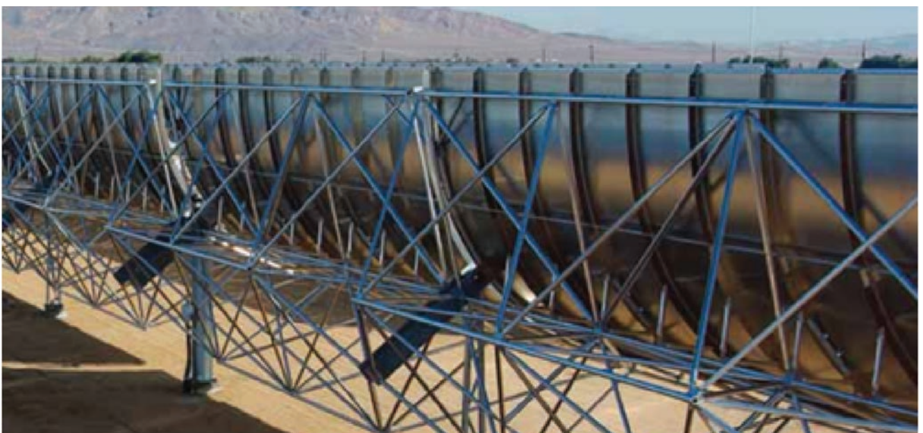
Figure 31: SkyFuel collector back structure and metal reflector sheets [20]
