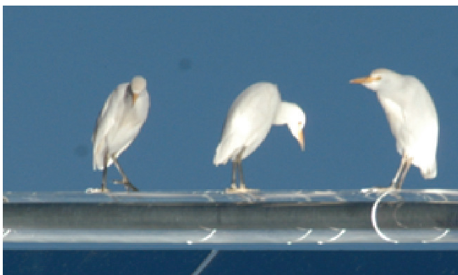
Figure 47: Thermal loss of current parabolic trough absorbers are low enough for birds to rest on the glass envelope (image © E. Lüpfer, CSP Services)
