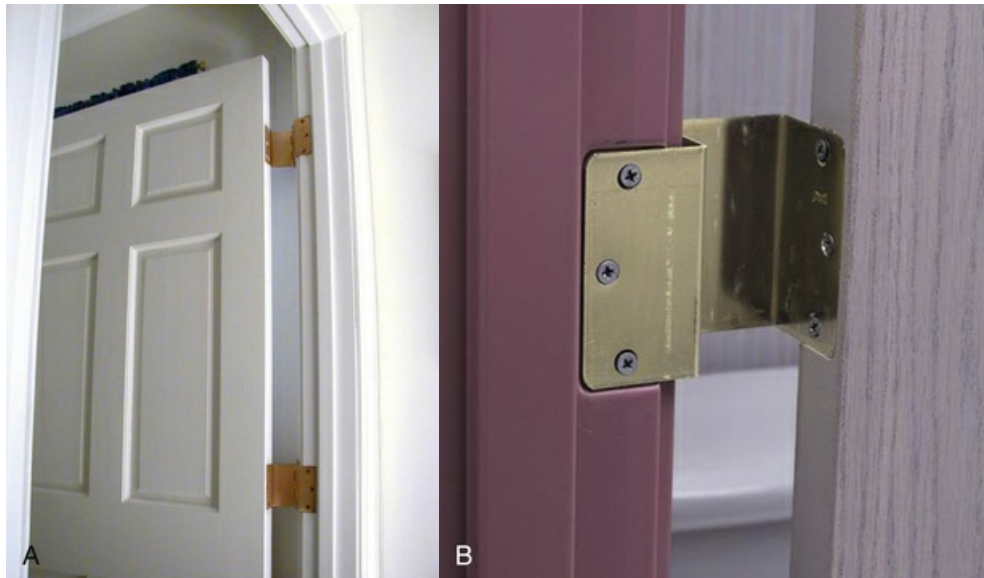
FIG 10.37 A, Offset door hinges allow for a wider doorway for wheelchair users. B, Close-up of offset hinges. (A courtesy How to Adapt: www.howtoadapt.com ; B courtesy Brigs Healthcare, West Des Moines, IA.)
