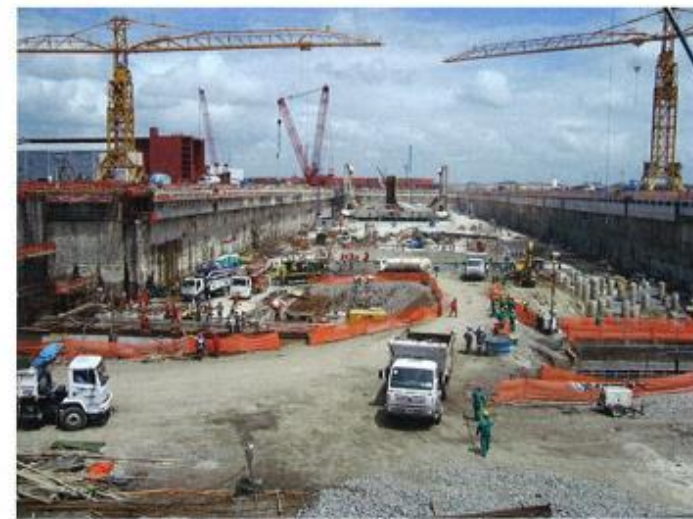
Construction underway for the dock floor
