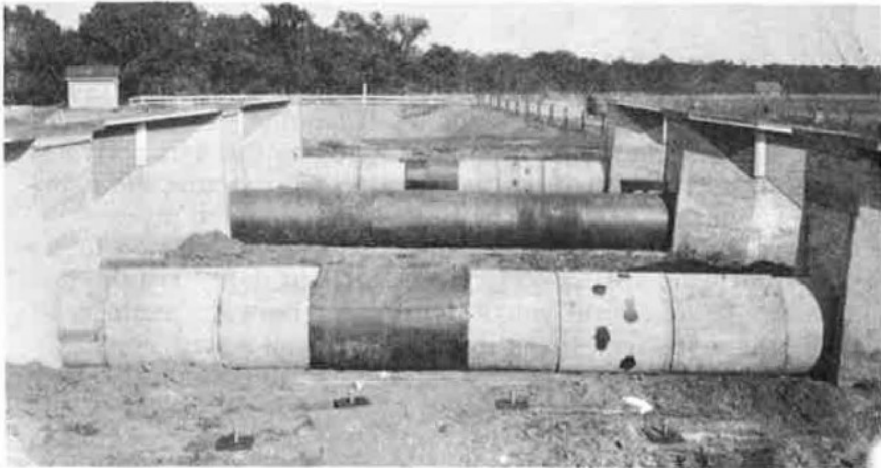
Figure 6. Experimental culverts before fill construction.
