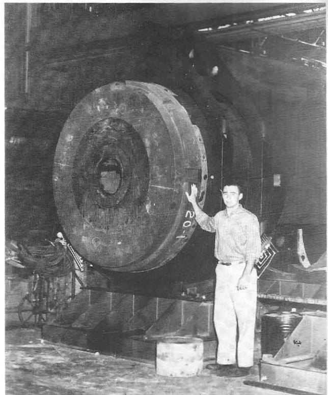
**FIGURE 42 – (Case B7) General view of a retaining ring forging, representing an external ring which is shrink fitted over the (dark) core of an extrusion chamber section. The chamber assembly comprises five adjoining rings.**
