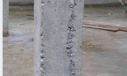
Figure 3.5 “Honeycombing” showing shoddy construction
