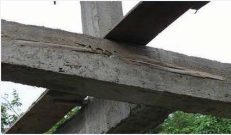
Figure 3.4 Debris embedded in a concrete support beam
