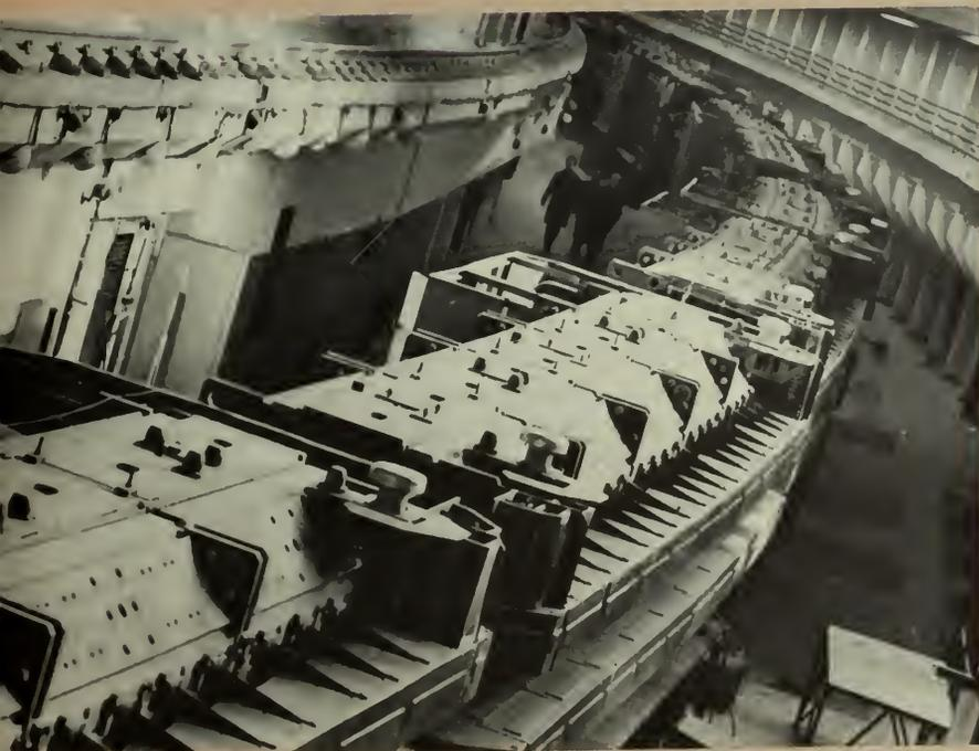
Russian nuclear physicists are doing important research at the two installations shown on this page. Above, is the 10 BeV capacity proton synchrotron accelerator located at the Dubna Joint Nuclear Research Institute. Below, is the proton synchrotron at Serpukhov which began operation in 1968. Its capacity is rated at 70 BeV.
