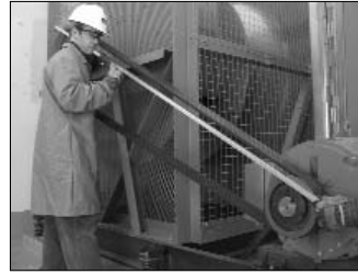
Using a straight edge to check alignment
