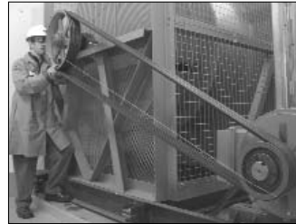
Using a string to check alignment
