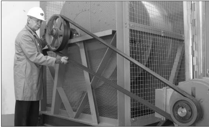
Begin by inspecting the belt
