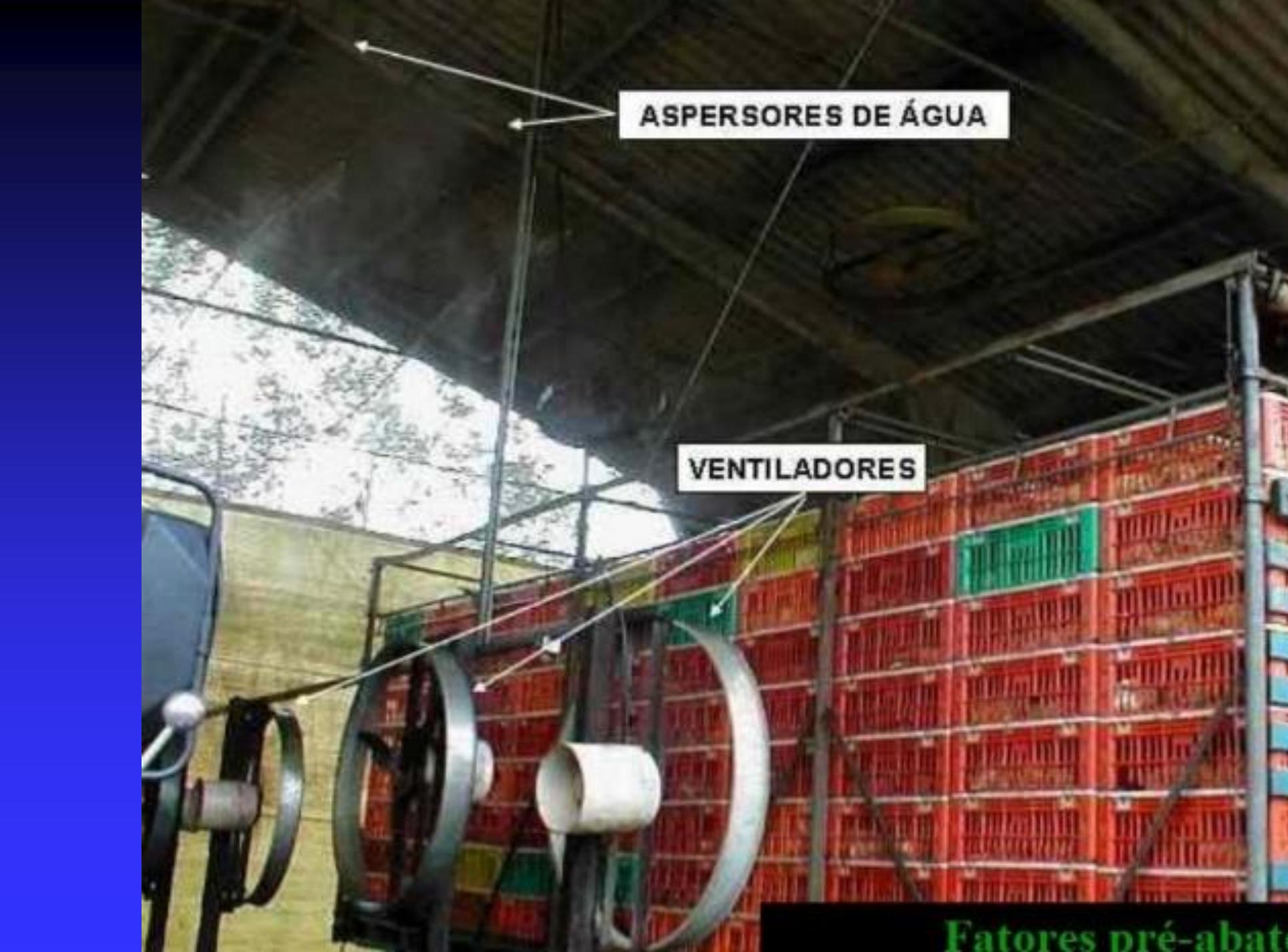
A photograph of a poultry processing facility. The ceiling is made of corrugated metal and has several water sprayers (aspersores) and fans (ventiladores) installed. The walls are lined with red plastic crates. A white box with black text points to the water sprayers, and another white box with black text points to the fans. The text 'Fatores pré-abate' is visible in the bottom right corner.
