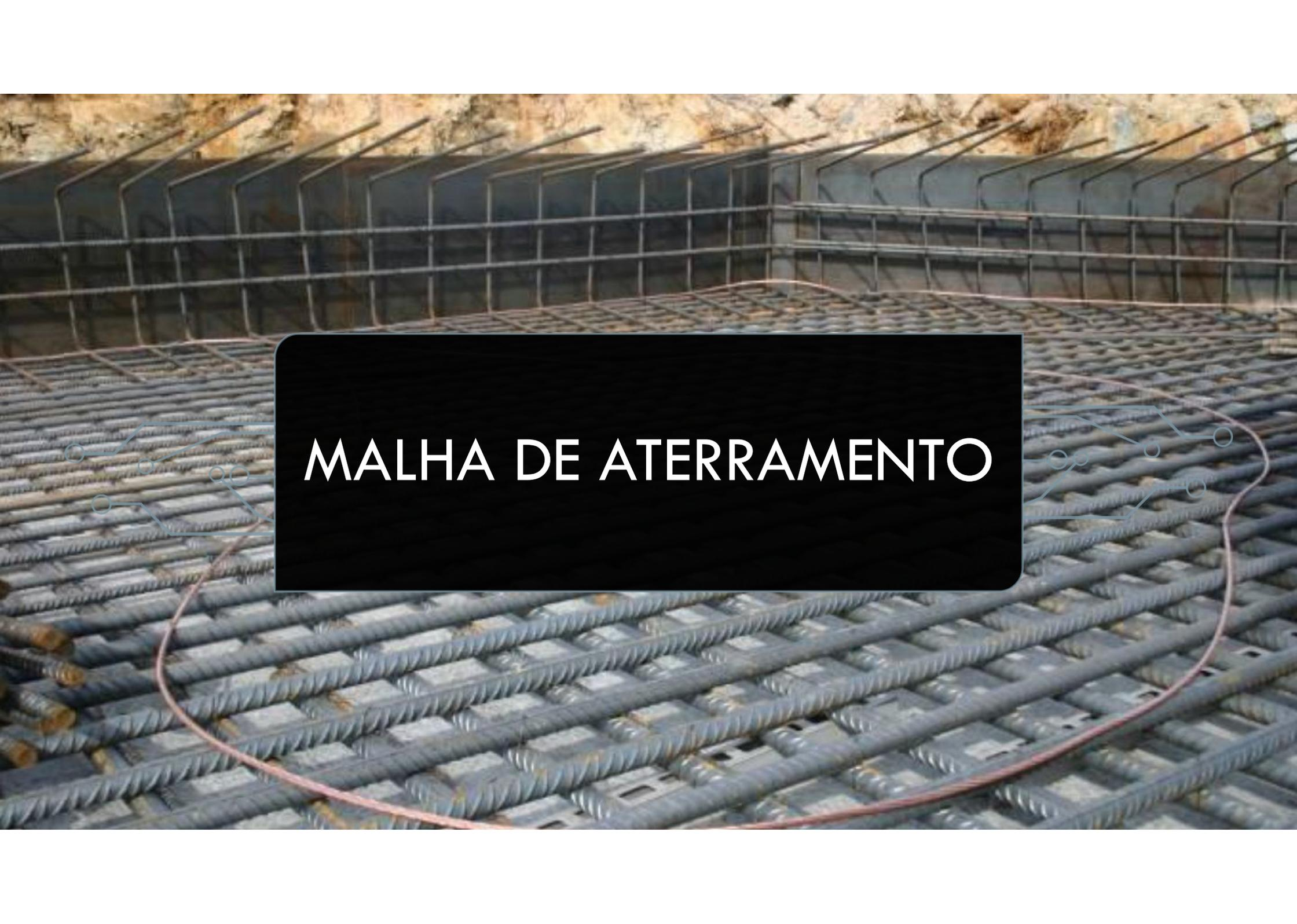
A photograph showing a construction site with a grid of steel reinforcement bars (rebar) laid out on a concrete slab. The rebar is arranged in a regular grid pattern, and the concrete is visible in the background. A black rectangular box with rounded corners is overlaid on the center of the image, containing the text "MALHA DE ATERRAMENTO".
