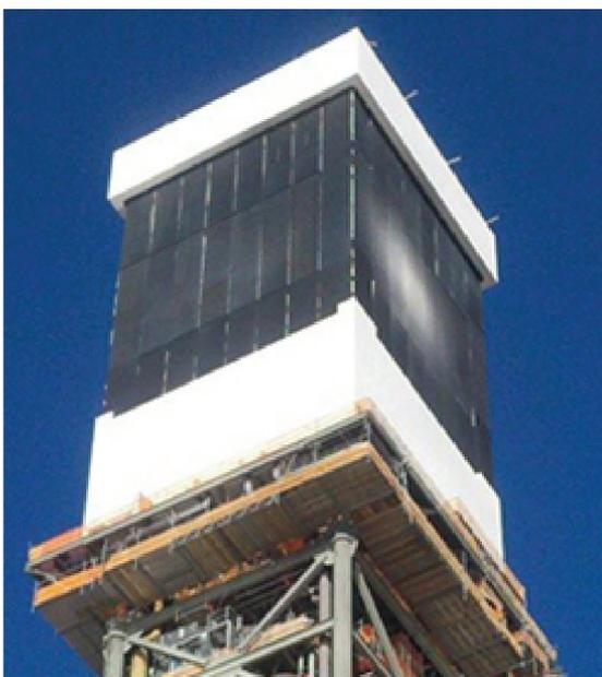
Figure 22: Brightsource external receiver (Ivanpah)
