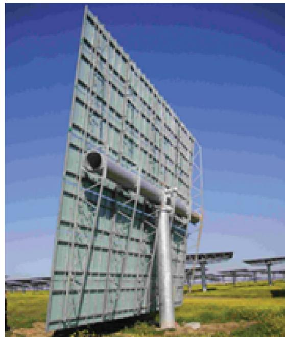
Figure 14: T-type heliostat with azimuth-elevation axis orientation
