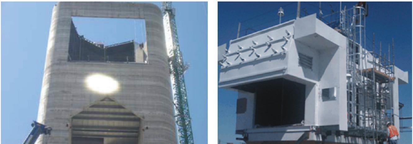
Figure 21: PS10 receiver during installation (left); double-cavity receiver (eSolar) (right)
