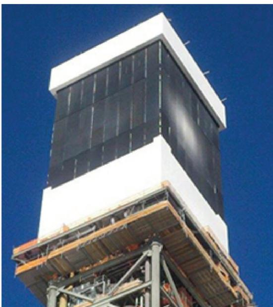
Figure 22: Brightsource external receiver (Ivanpah)
