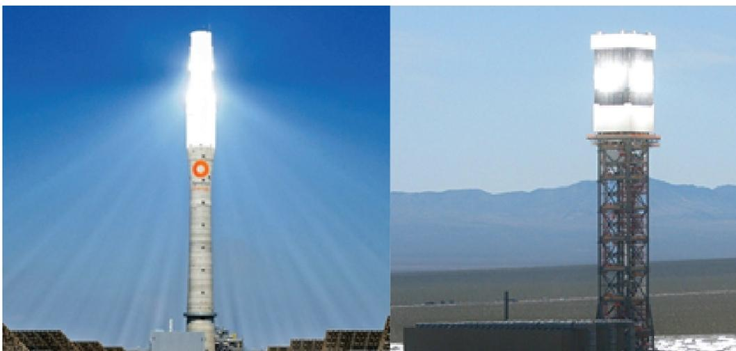
Figure 25: Examples of existing tower constructions (left: concrete tower, right: steel tower)
