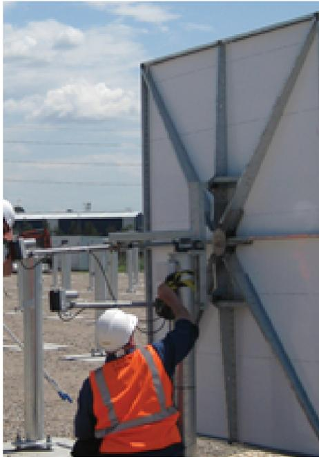
Figure 17: Heliostat with two linear drives and horizontal first axis [13]
