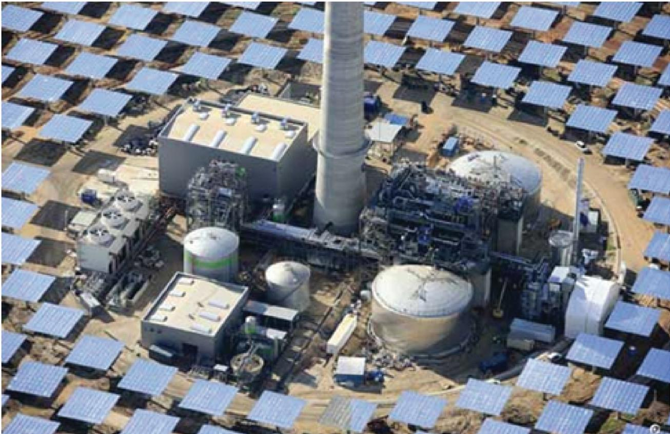
Figure 27: Thermal storage of Gemasolar plant (two tanks right of tower; 15h capacity)
