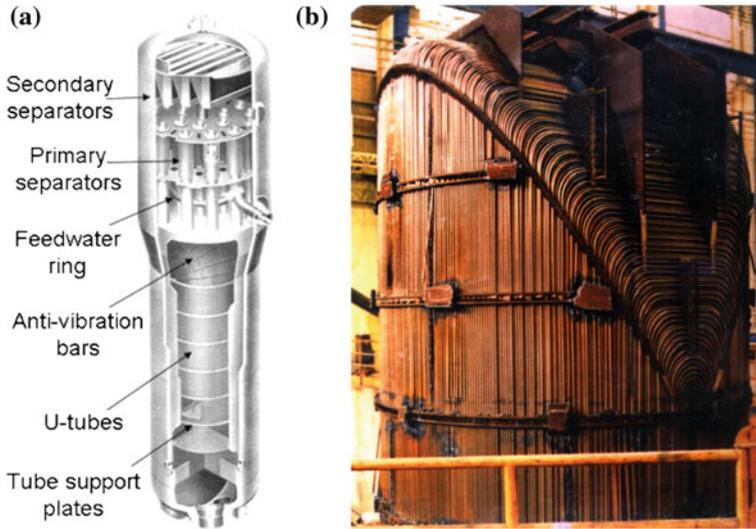
**Fig. 3.16** Steam generator top view of an old steam generator from a nuclear power plant (Source [56]). The left figure shows a new modern steam generator for comparison (Source [57]). **a** Advanced steam generator. Copyright: Mitsubishi Heavy Industries **b** Old steam generator (with permission of US-NRC)
