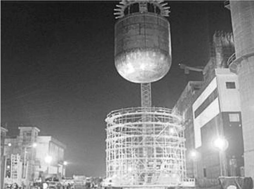
**Fig. 3.4** Installation of the main vessel of India's prototype fast breeder reactor, PFBR (copyright 2011 Nuclear Engineering International magazine, [www.neimagazine.com](http://www.neimagazine.com))
