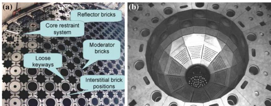
**Fig. 3.15** Graphite cores of gas cooled reactors, advanced gas reactor (AGR) [54] and high temperature reactor [55]. **a** with the permission of B. Marsden (Manchester) **b** with the permission of Y. Sun, INET
