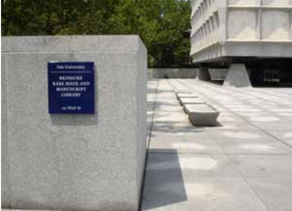
Recessed glass entrance; sign placed on nearby wall.
