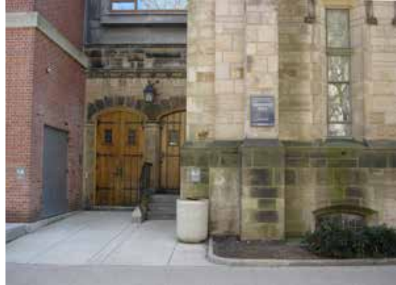
Sign placed above projecting ledge of "base."
