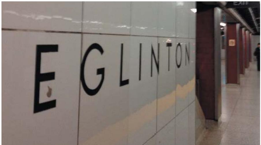
Figure 8. Original station identification signage engraved directly into Vitrolite tile panel at subway platform level.
