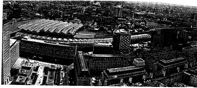
3.22: The International Terminal Waterloo by Nicholas Grimshaw & Partners. Source: James Pole.
