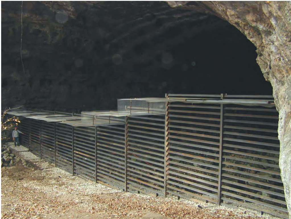
FIGURE 3 A large half gate or fly-over at Great Spirit Cave, Missouri, completed in 2002. The gate weighs 18 metric tons and measures 31 m wide by 5 m high. It protects gray bats ( Myotis grisescens ) in summer, Indiana bats ( Myotis sodalis ) in winter, and multiple resources in this Natural Area cave.
