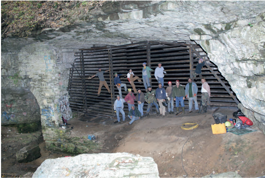
FIGURE 2 The National Cave Gating Workshop, 2009, built a bat-friendly, full cave gate at Cliff Cave, Missouri, to protect multiple resources, including endangered Indiana bats.
