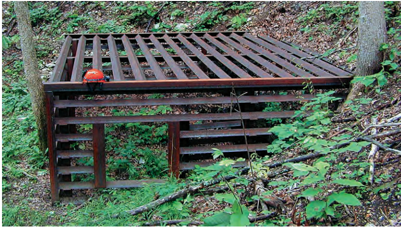
FIGURE 4 A cupola or cage gate over a sinkhole entrance, which allows bats to gain altitude and exit laterally, easier than flying up through a horizontal grate.
