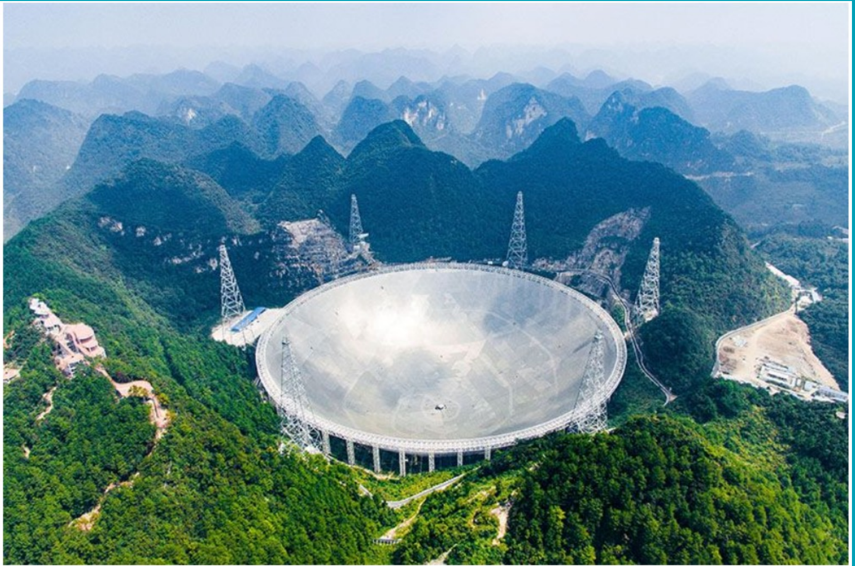
The world's single largest radio telescope. Completed in 2016, the 500 meter Aperture Spherical Radio Telescope (FAST)
