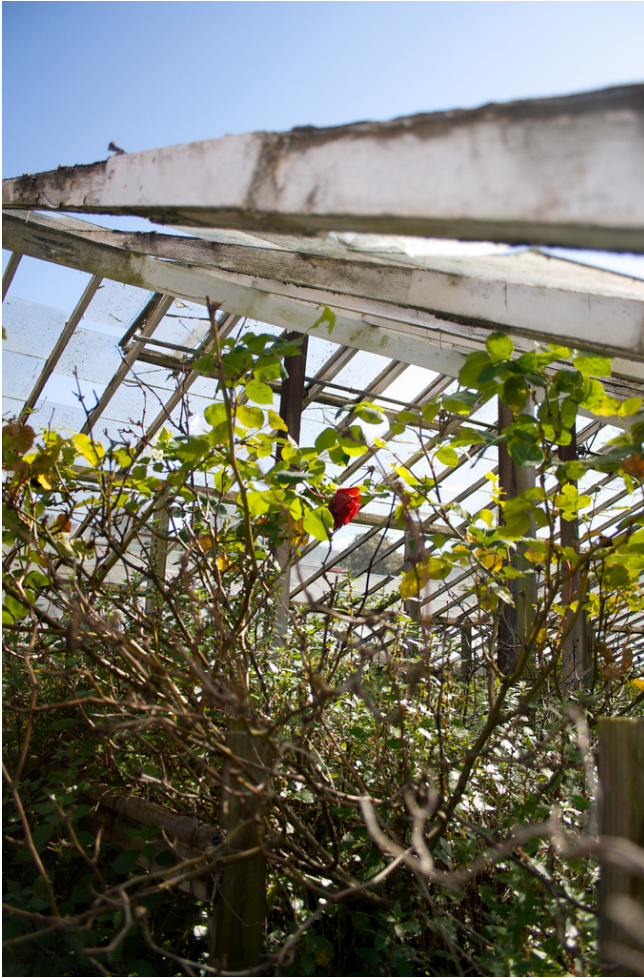
Greenhouse built from reclaimed materials
