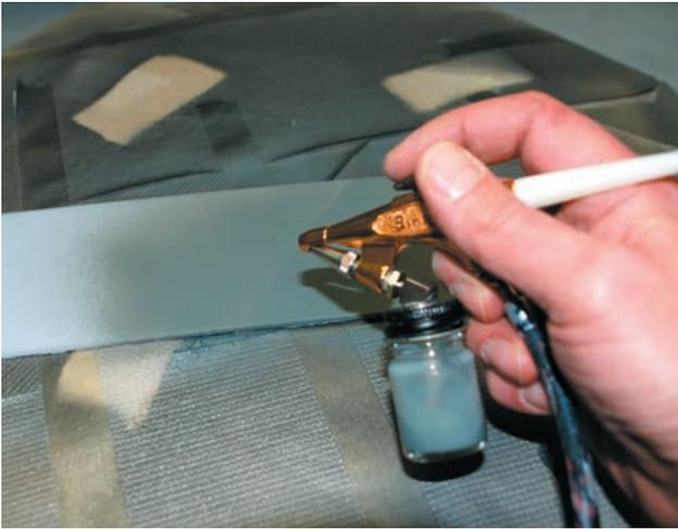
**Step 3** The airbrush is now hooked up to the compressor (20–40 PSI) and tested on a scrap piece of plastic in the spray booth. The nozzle flow is adjusted and if the paint is not flowing, more airbrush medium will be added.
