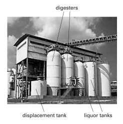
Figure 1.5. Batch-wise cooking configuration employing two digesters and accompanied with tanks for liquor and pulp (Metso Paper).
