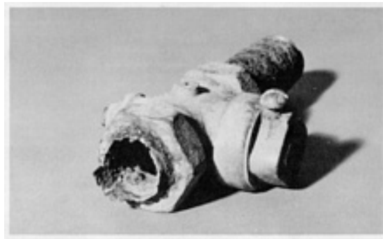
Fig. 13 Galvanic corrosion of steel pipe at brass fitting in humid marine atmosphere. Courtesy of R. Baboian, Texas Instruments, Inc.
