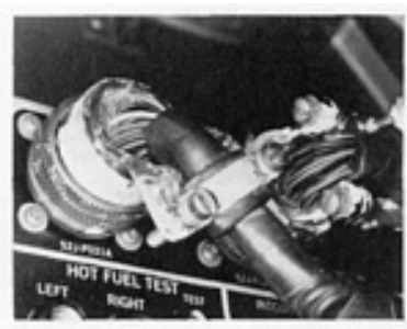
Fig. 17 Corroded low-voltage electrical connector on avionic equipment
