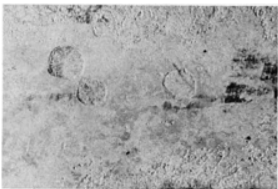
Fig. 62 Circular areas of corrosion observed directly overhead in a UNS NO8904 steaming tube due to formation of acidic condensate drips. Approximately \frac{3}{4} \times
