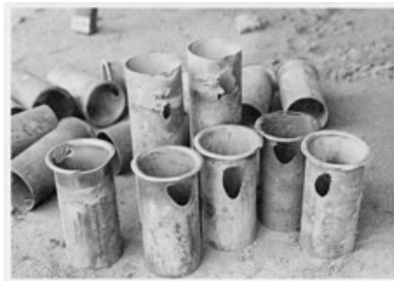
Fig. 5 Eroded tube inserts from the inlet end of a fire-tube boiler. The inserts were eroded by particle-laden flue gas, which was forced to run as it entered the boiler.
