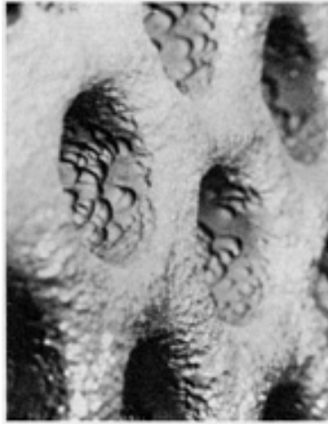
Fig. 9 Erosion-corrosion of carbon steel tubes in a closed feedwater heater. Courtesy of the Electric Power Research Institute
