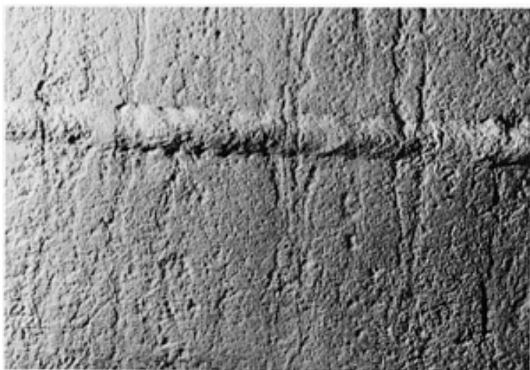
Fig. 61 Acidic condensate corrosion runs observed across a longitudinal seam weld on the wall of a UNS NO8904 steaming tube (see Fig. 56 left side wall)
