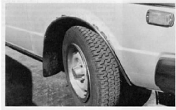
Fig. 12 Galvanic corrosion of painted steel auto body panel in contact with stainless steel wheel opening molding. Courtesy of R. Baboian, Texas Instruments, Inc.
