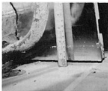
Fig. 8 Crevice corrosion of a type 316L checking plate located adjacent to a headbox apron. Corrosion developed under pulp pads that formed despite the highly polished surface.
