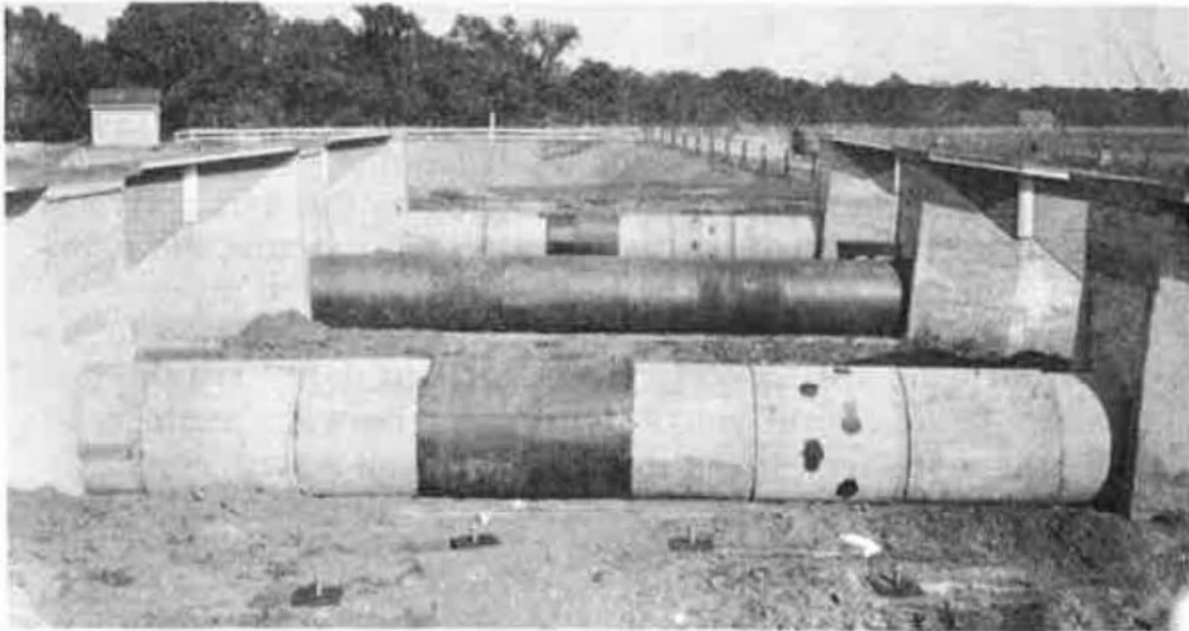
Figure 6. Experimental culverts before fill construction.
