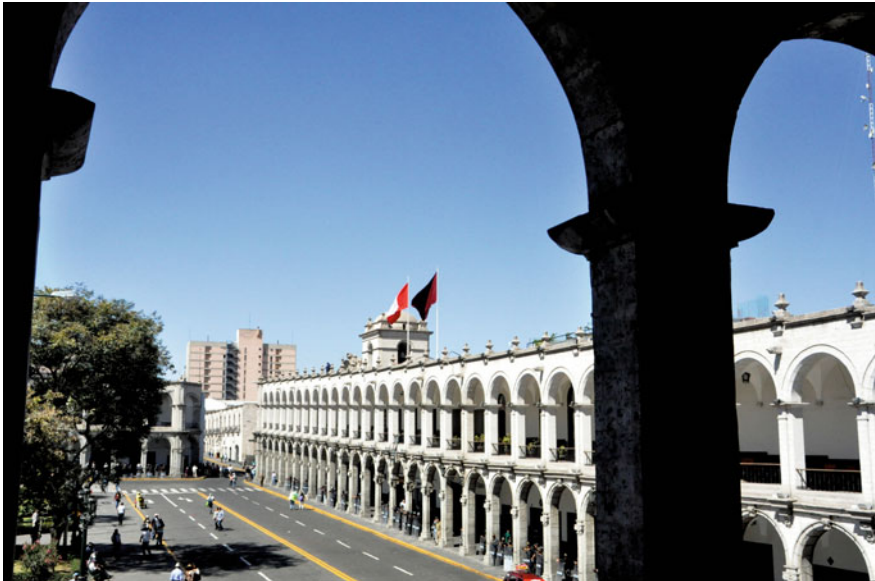
Fig. 6.13 Impressive historical buildings in the main square of Arequipa built with white volcanic rock blocks Credit Menegat and Fontana
